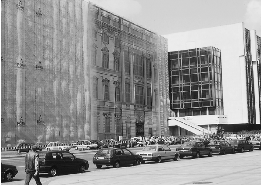
Figure 6.11 Palast der Republik (Palace of the Republic), Heinz Graffunder and Karl-Ernst Swora, 1973–76, Berlin, and temporary reconstruction of Schloss (Palace), 1993
