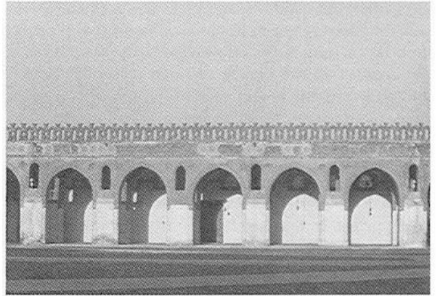
Pl. 40. Side arcade at the mosque of Ibn Ṭulūn.
