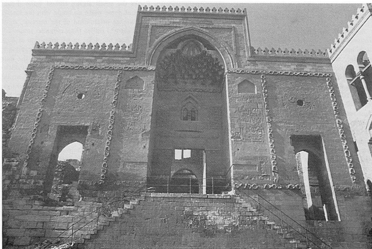
Pl. 100. The facade of the hospital of Sultan al-Muʿayyad.
