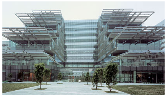
The building is designed like a leaf that transforms sunlight into energy. A series of south-facing terraced gardens is home to thick vegetation and more than 1,000 square metres (10,764 square feet) of photovoltaic panels that provide a substantial amount of the building's energy requirements. The horseshoe shape is in juxtaposition with the sun's movements, thus allowing for continuous natural illumination of the offices and reducing energy requirements.
