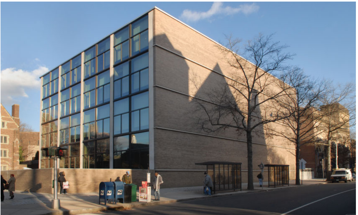
A sunken court on the corner of York and Chapel Streets has been reopened in the renovation which also replaced the curtain walls on the west and north sides. On the south, a solid brick facade defers to the building's neighbours in historical styles.
