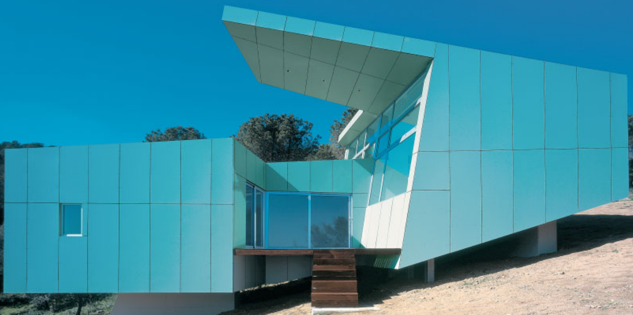
Fabrizio Leoni Architettura with Olindo Merone Architetto, O House, Capoterra, Cagliari, Sardinia, 2004 This house, located in dense terrain, uses an extremely innovative approach based on the chassis of an automobile.
