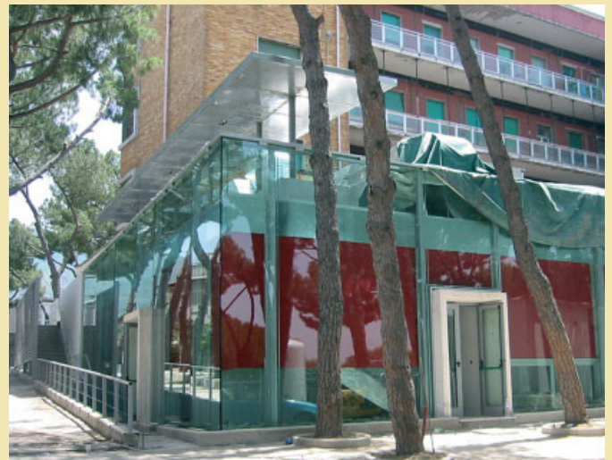
Vulcanica Architettura, Addition, renovation and new operating wing, Nostra Signora di Lourdes Clinic, Massa di Somma, Naples, 2003 A transparent box of glass and steel elements wraps around the existing volume.
