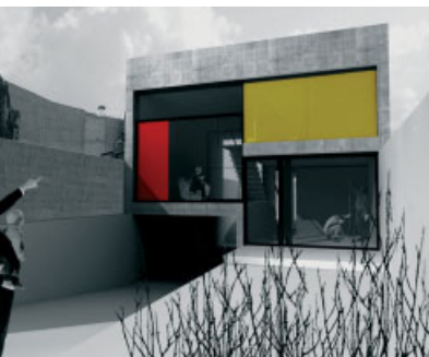
Maria Giuseppina Grasso Cannizzo, RGV House, Vittoria, Sicily, 2006 Here, two volumes in reinforced concrete, with independent structures, organise interchanging spaces. The house has four levels with a total height of less than 6 metres (19.7 feet).
