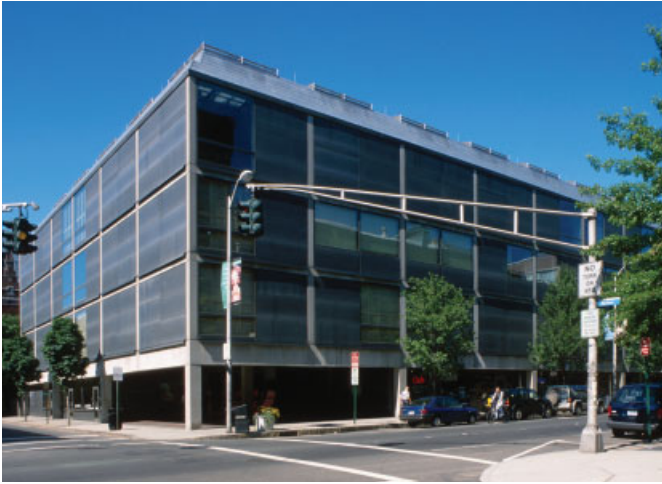
Kahn's last major building in the US faces the Yale University Art Gallery across Chapel Street, but it is sheathed in unpolished, dark stainless-steel panelling and glass, inserted within a smooth concrete structural grid. The entrance is tucked into a void on the southeast corner (shown here) where it leads to a four-storey skylighted courtyard, expressed by a break in the grid on the facade.
