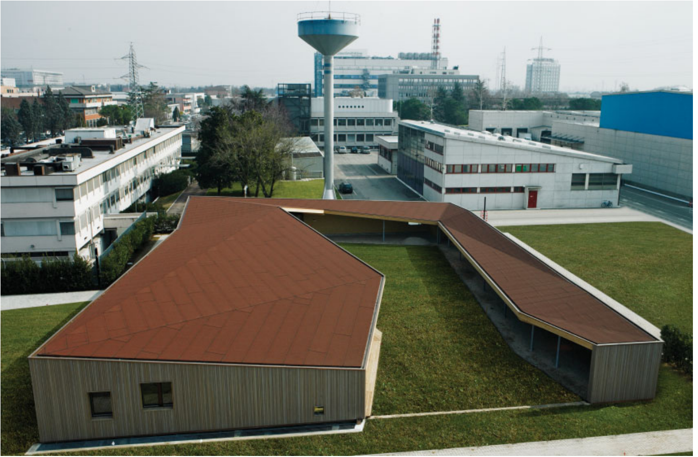
Antonio Citterio, Nursery School for a multinational pharmaceutical company, Verona, 2005 Aerial view of the nursery showing the volume of the classrooms, the portico and interior courtyard.
