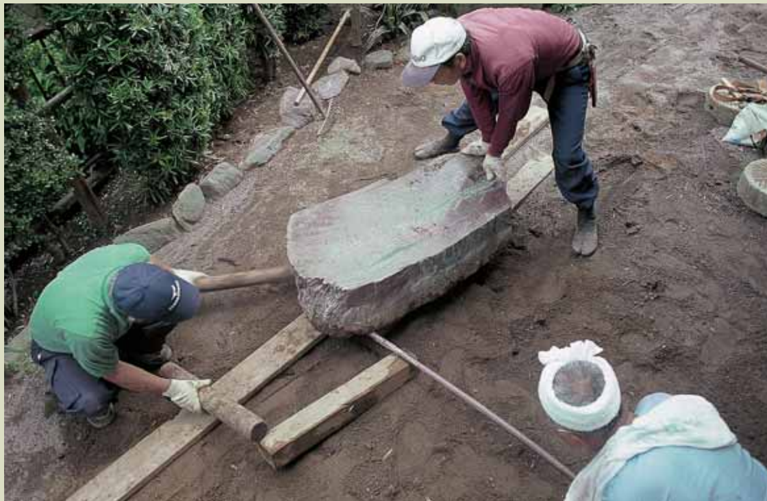
ABOVE Moving a heavy stone in a private garden by traditional methods, using wood rollers, planks and plenty of muscle.
