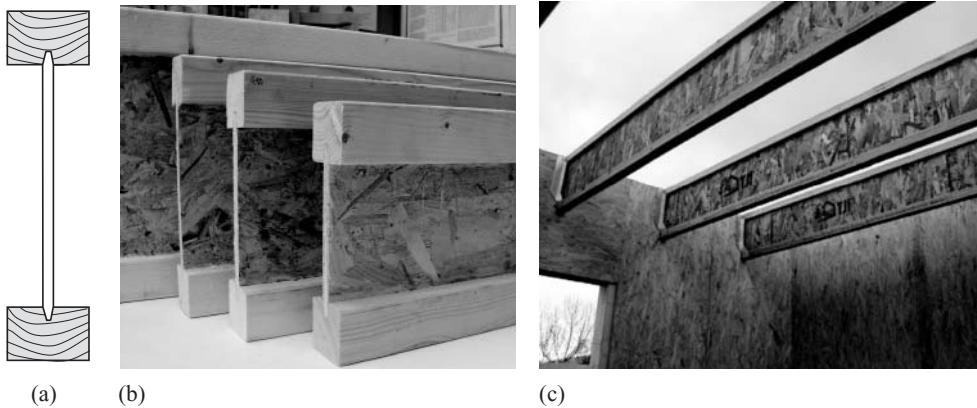
Fig. 1.15. Typical I-joists and their application.
