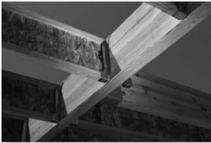
(a) I-beams floor joists
