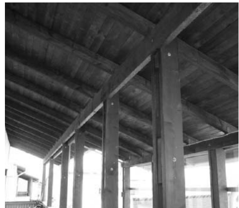
(b) Bolted spaced columns with solid sections
