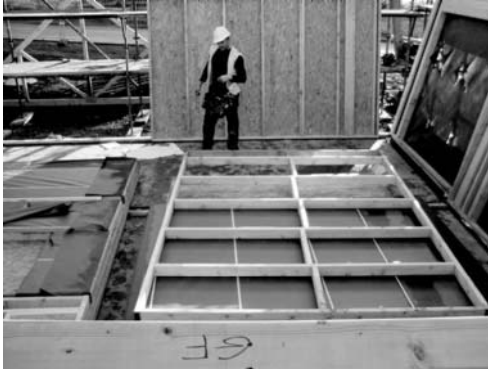
(a) Timber wall during assembly and erection
