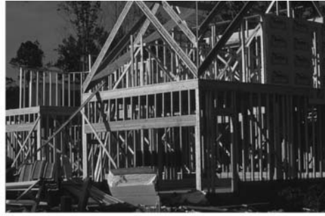
(b) I-beams in sloped roofs (photo courtesy of APA, The Engineered Wood Association)
