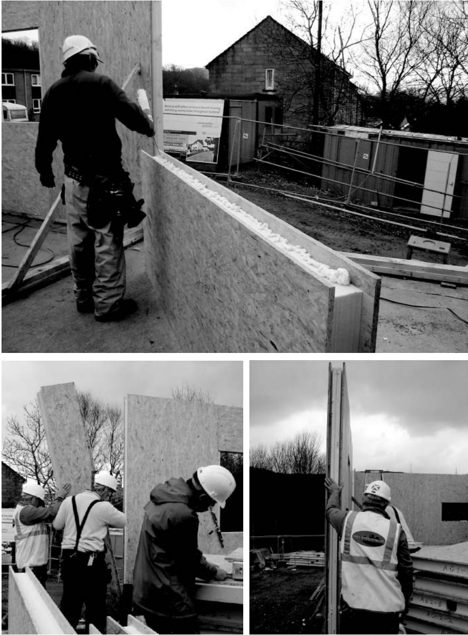
Fig. 1.17. SIPs during construction.
