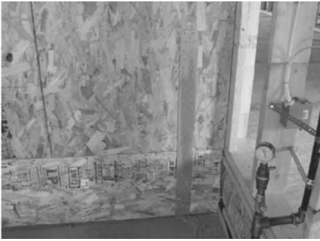
(a) Nailed holding-down strap
