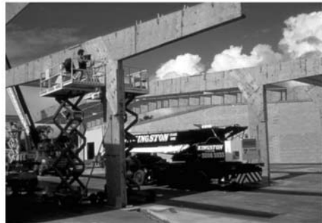
(f) Large span box portal frames using LVL (photo courtesy of Engineered Wood products Association of Australia (EWPAA))
