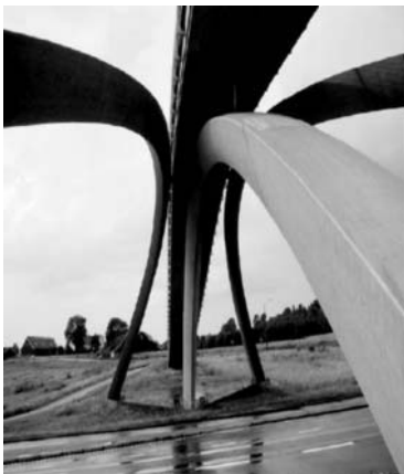
(g) Footbridge (photo courtesy of Engineered Wood Products Association of Australasia (EWPAA))
