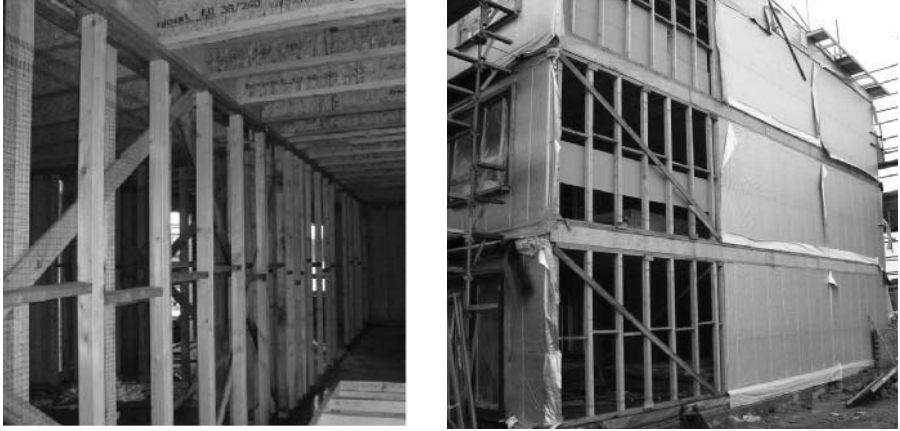
Fig. 5.15. Stud walls during construction.
