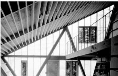
(c) Deep long-span LVL joists exposed
