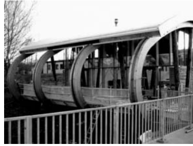
(b) Curved structure (photo courtesy of Constructional Timber Limited, a member of the Glued Laminated Timber Association, UK)
