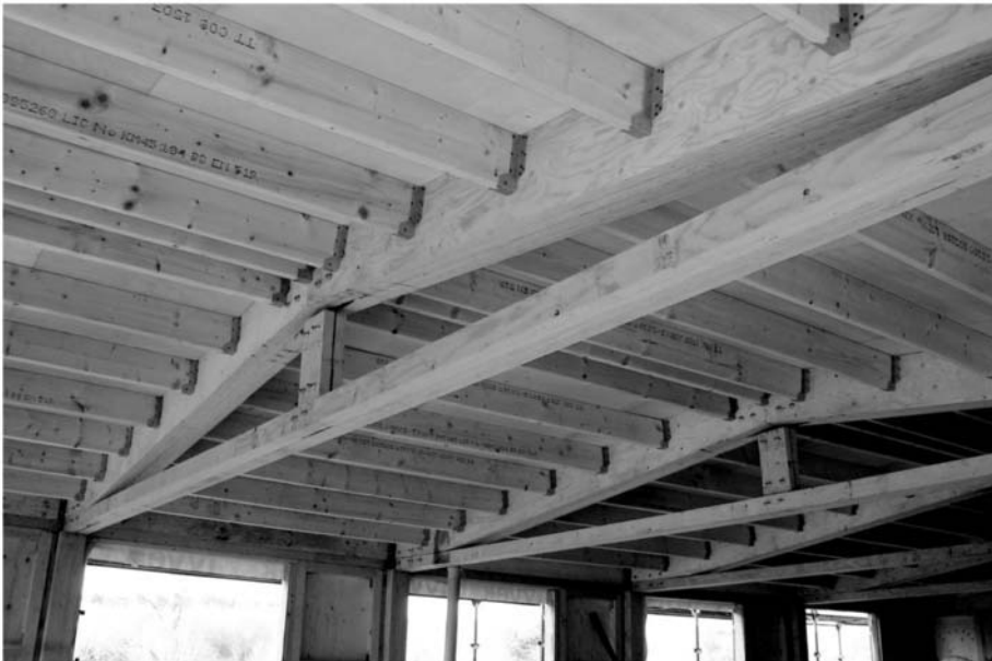
(c) LVL truss members (Cullen Building Products' HQ during construction)
