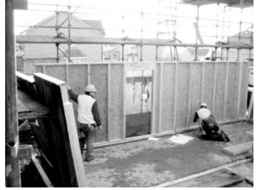
(a) Timber wall during assembly and erection
