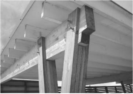
(c) Bolted timber-to-timber connection
