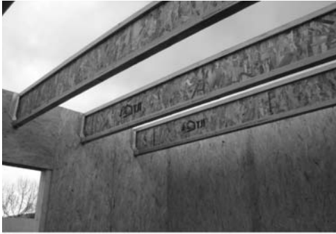
(a) I-beams floor joists
