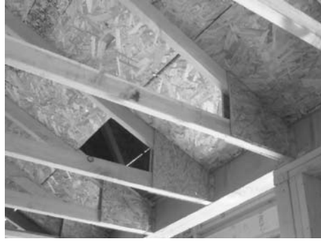
(b) Nailed OSB gusset joints
