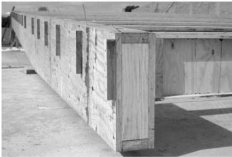
(e) Large span box beam and I-joists using LVL (photo courtesy of Engineered Wood products Association of Australia (EWPAA))
