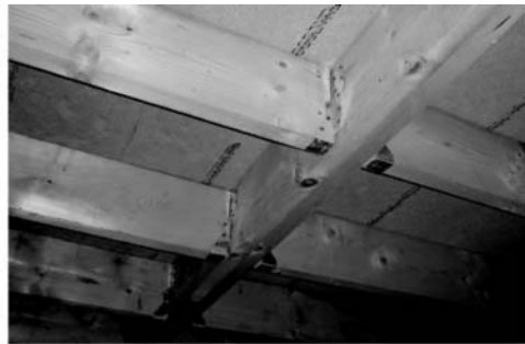
(b) Solid section trimmer beam and joists
