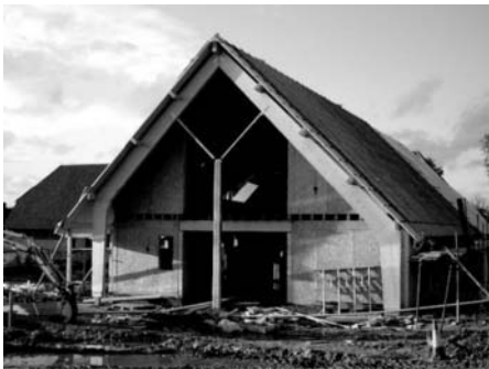
(e) Portal frame (photo courtesy of Constructional Timber Ltd, a member of the Glued Laminated Timber Association, UK)
