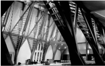
(c) Sloped columns (photo courtesy of APA, The Engineered Wood Association)
