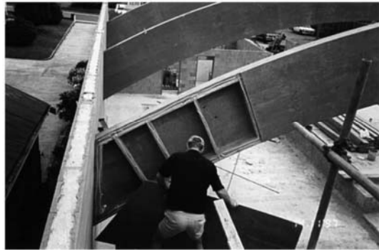
(d) Curved box beam (photo courtesy of Fred Bosveld and Peter Yttrup)
