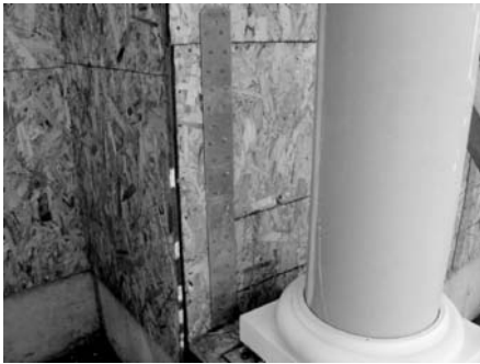
(b) Holding-down strap to prevent overturning
