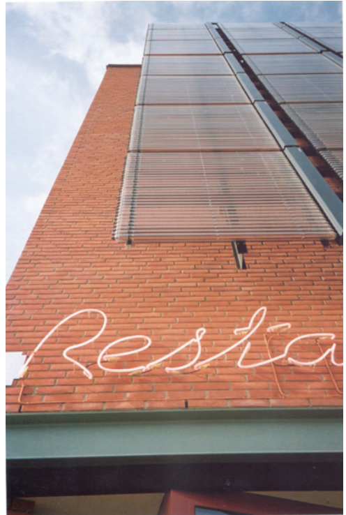
Figure 15.2 Solar collectors operated by Sydcraft, a district energy supplier on the Tegelborden block on the Sundspromenaden (architect: Mansson Dahlback; photograph: Christopher John Hancock)
