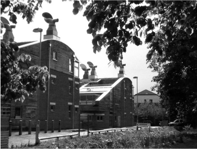
Figure 15.13 Completed project west elevation
