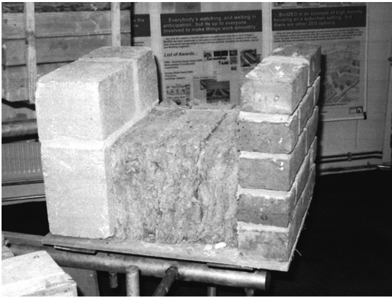
Figure 15.15 Masonry wall construction (courtesy of Bill Dunster)
