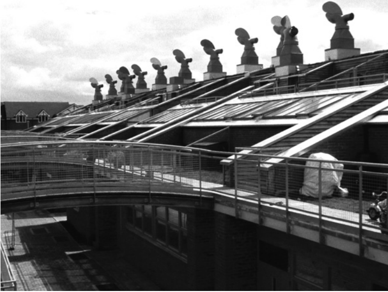
Figure 15.14 South elevation with work spaces at ground level and roof gardens serving dwellings opposite
