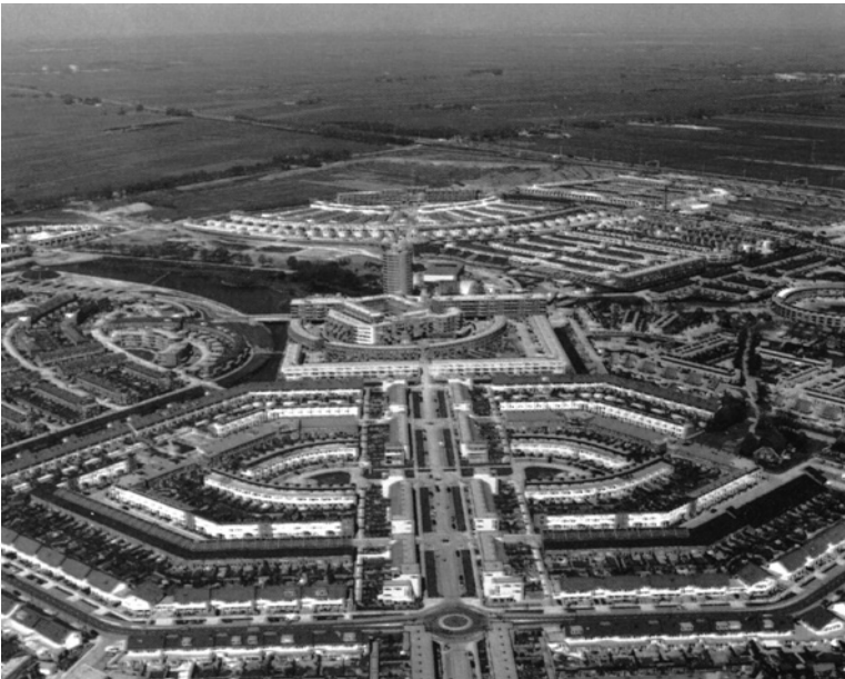
Figure 6.3 The new town of Nieuwland near Amersfoort (courtesy of Ecofys and REW)
