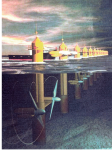
Figure 11.13 Tidal stream turbines or tidal mills, serviced above water (courtesy of Marine Current Turbines (MCT))
