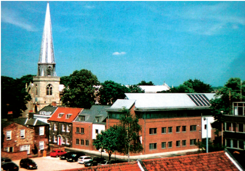
Figure 15.10 Borough Council offices, King's Lynn, Norfolk (courtesy of Ecotech)
