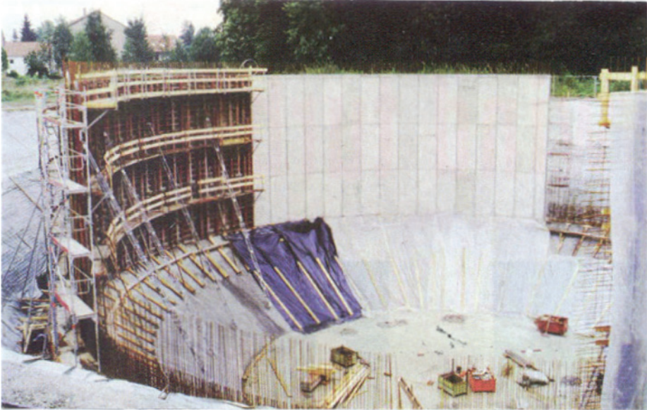
Figure 2.12 Seasonal storage tank under construction, Friedrichshafen (courtesy of Renewable Energy World )
