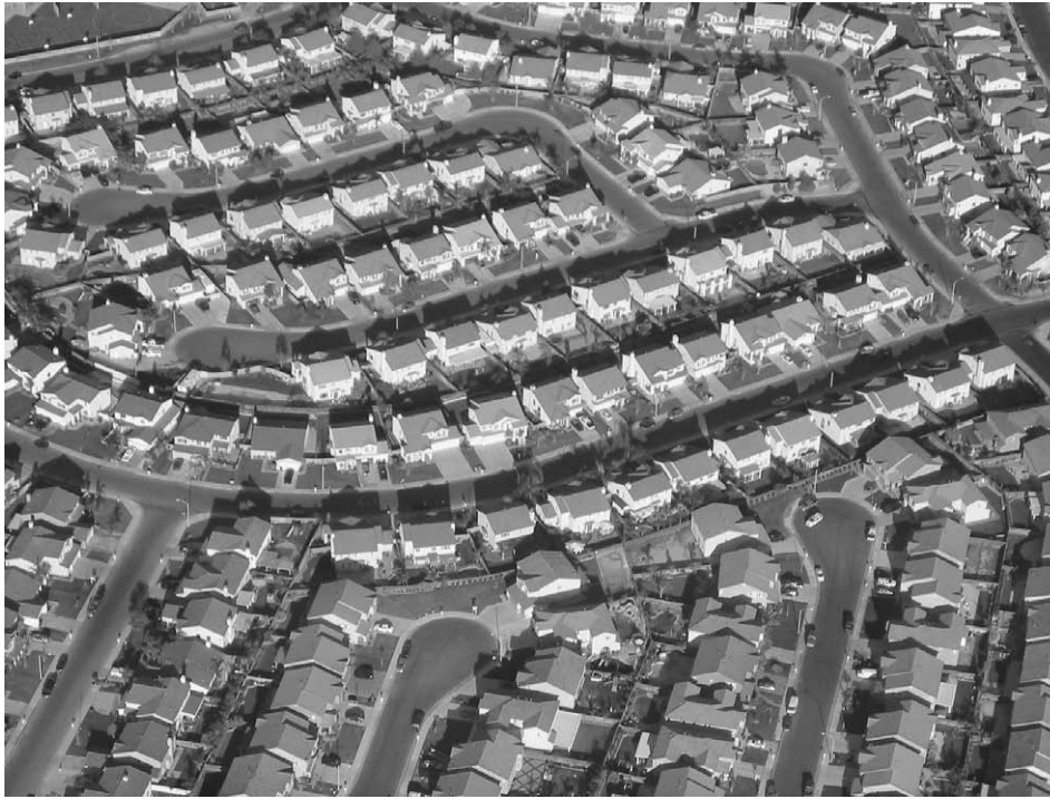
Figure 6-3 The Subdivision Energy Analysis Tool can analyze energy impacts for different neighborhood and street layouts. Jon Roberts
