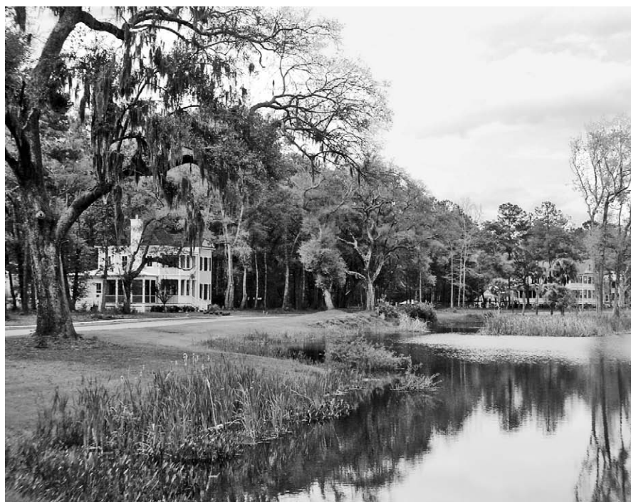
Figure 7-2 Habersham's constructed wetland filters stormwater before it drains to creeks and marshes. Duany Plater-Zyberk and Company, Charlotte, NC
