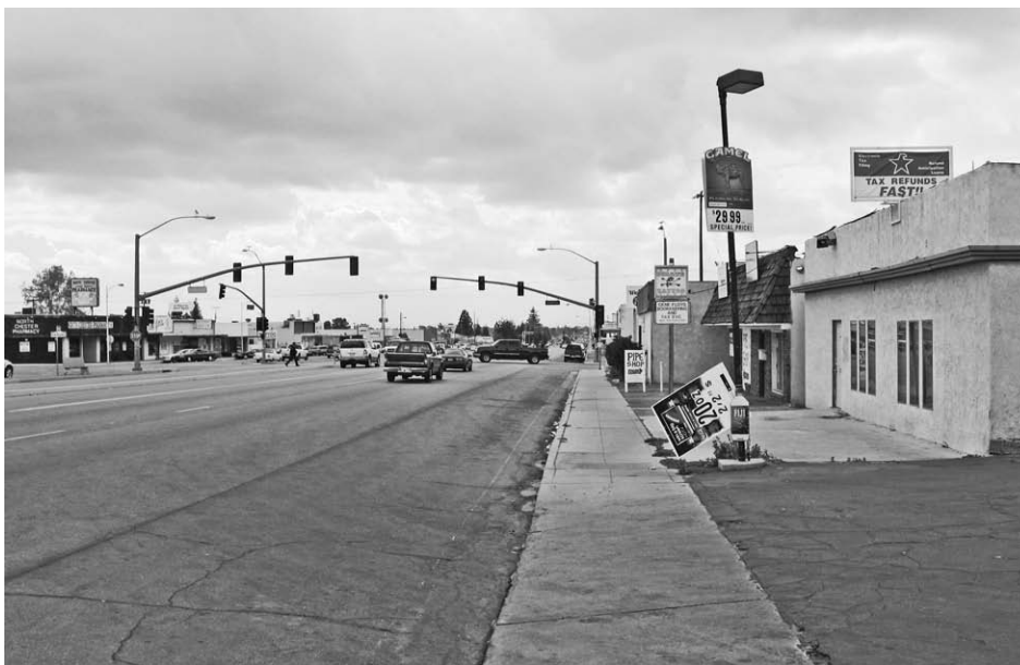
Figure 1-16 Throughout the country, thousands of deteriorating, auto-dominated corridors require conversion into “complete streets” or multi-use places. Stephen Coyle
