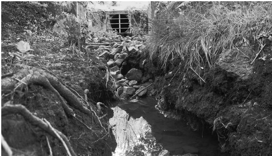
Figure 1-19 Conventional stormwater infrastructure often channels runoff rather than managing the water for reuse or recharge. UCSC Storm Water Management Program Environmental Health and Safety Department
