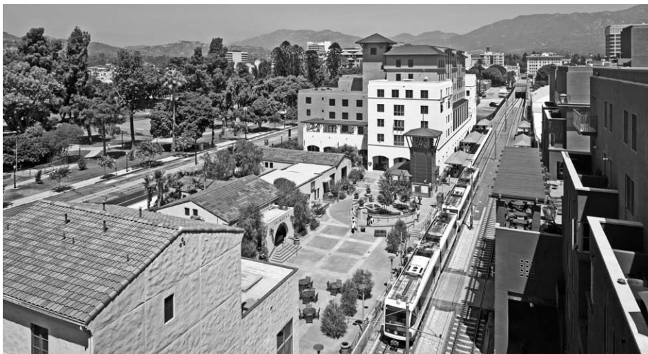
Figure 1-24 Del Mar Station designed by Moule Polyzoides Architects and Urbanists represents a pedestrian- and transit- oriented development. Tom Bonner Photography
