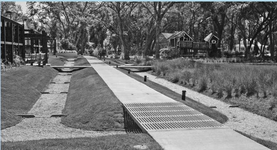
Figure 7-5 During fair weather at Habersham, the same gravel swale is still an attractive feature with charming wooden footbridges. Duany Plater-Zyberk and Company, Charlotte, NC
