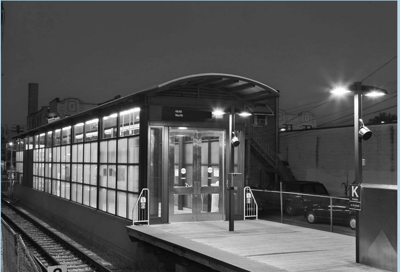
Figure 5-12 The Kedzie Station on the CTA Brown Line in Chicago, designed by Muller & Muller, Ltd., supports transit-oriented development. Congress for the New Urbanism
