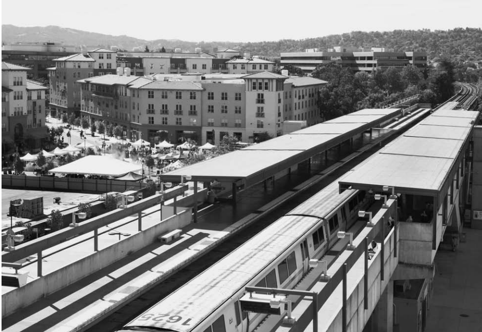
Figure 2-18 California's Contra Costa Centre/ Pleasant Hill BART Transit Village, the implementation of the second phase of a resilient, transit-oriented develop- ment. Doug Johnson, MVE & Partners, Inc., Architects
