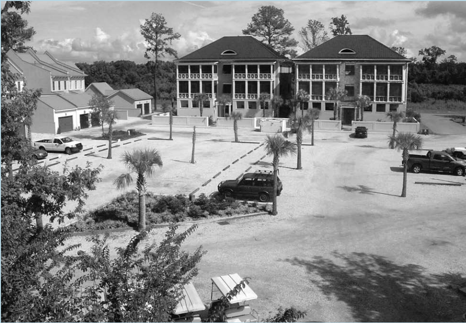
Figure 7-6 As a light imprint technique, the pervious parking plaza at Habersham reduces pavement required while it stores and filters stormwater. Duany Plater-Zyberk and Company, Charlotte, NC
