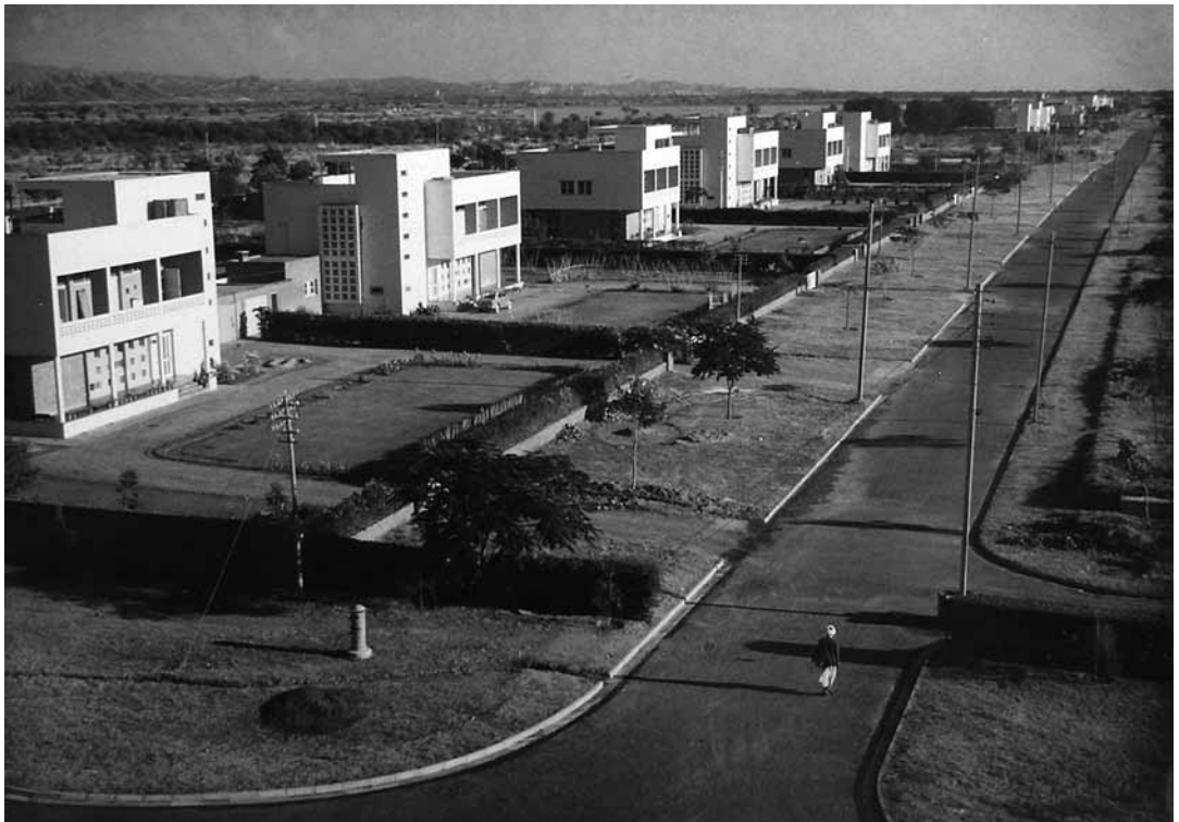
6.3 Large villas designed by Fry and Drew in sector 4, 1954
