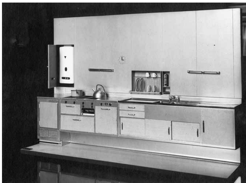
3.15 Kitchen Side of a Kitchen- Bathroom Unit, Kitchen Planning Exhibition, 1945
