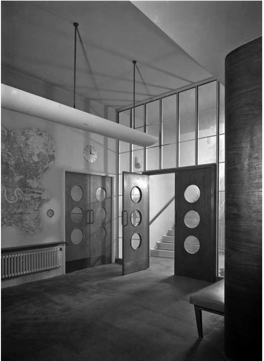
2.24 Entrance Hall, Cecil Residential Club, London, 1940
