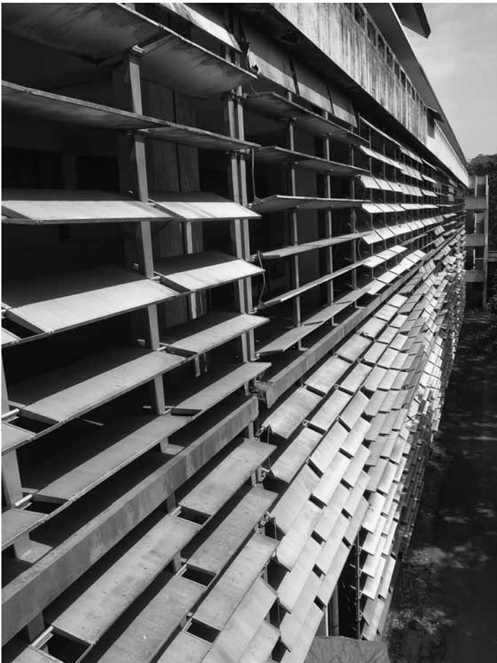
6.23 Government Press Building, Climatic controls, 2012
