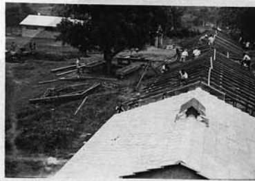
Erecting prefabricated trusses.
