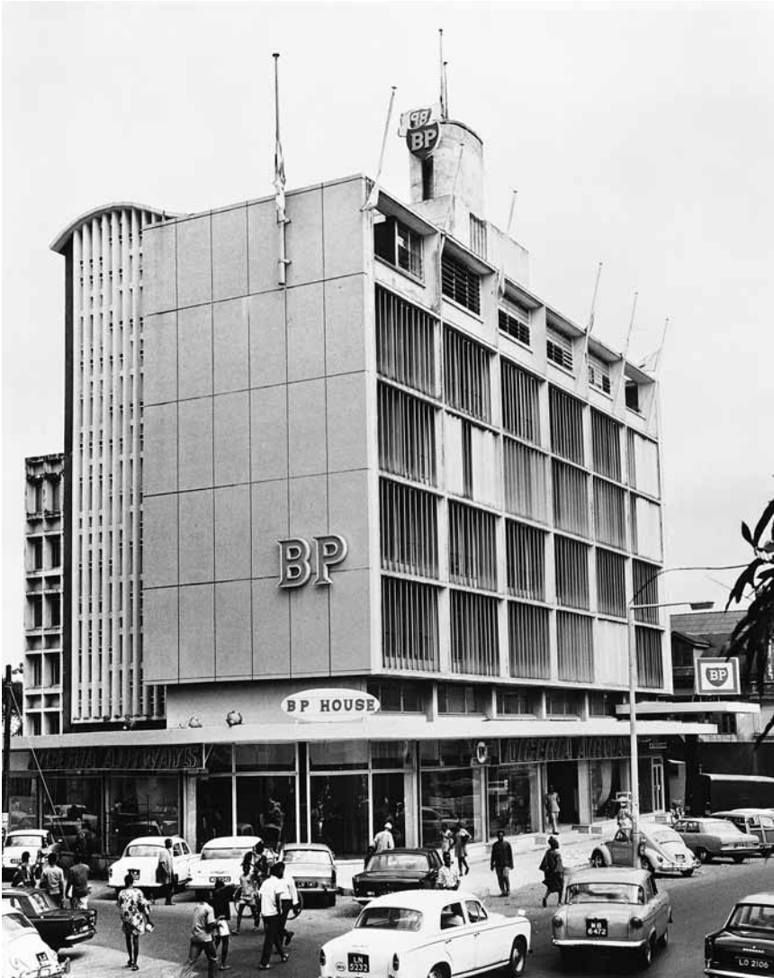
6.49 BP Offices, Lagos, 1962 Reproduced from the BP archive. © BP Plc
