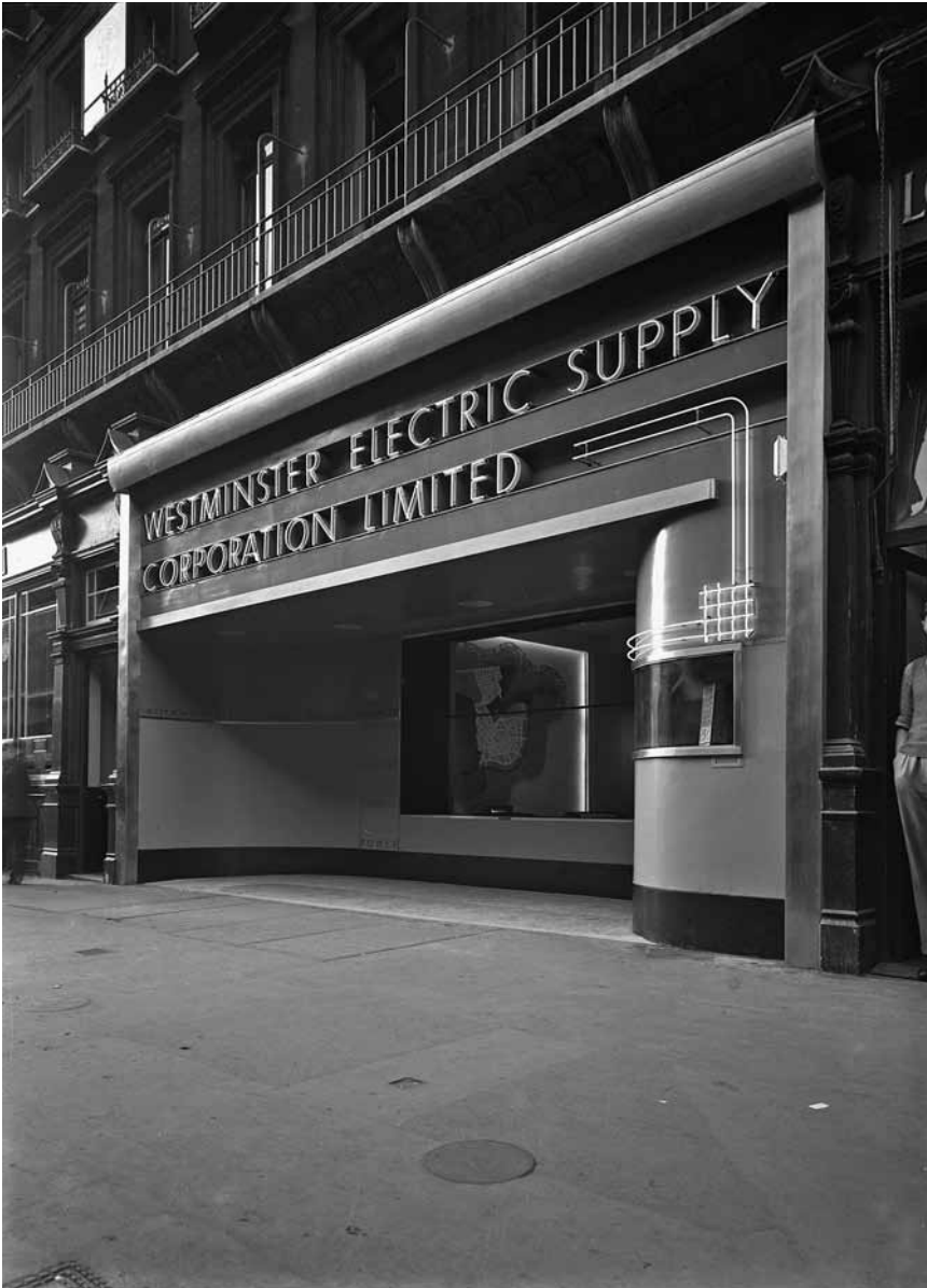
2.25 Westminster Electric Supply Corporation Showrooms, Victoria Street, London, 1933
