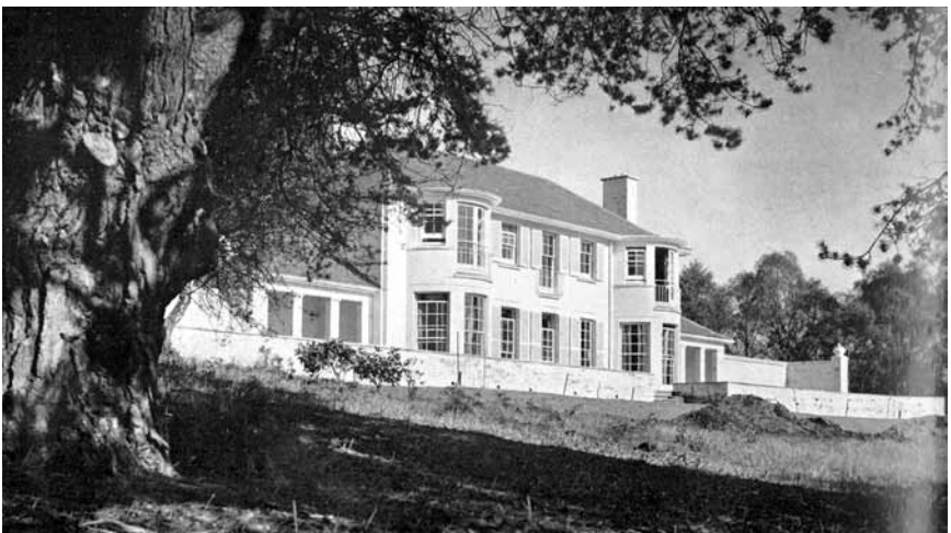
1.14 South Façade, Ridge End, Virginia Water, Surrey, 1932
