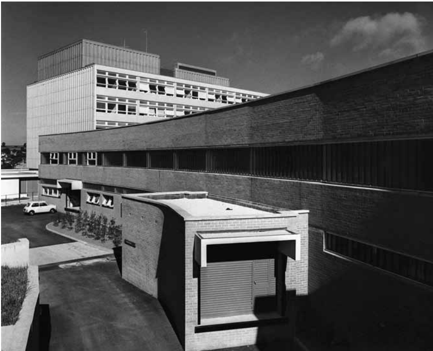
7.23 Theatre with pharmacy block to rear, Torbay Hospital, 1970
