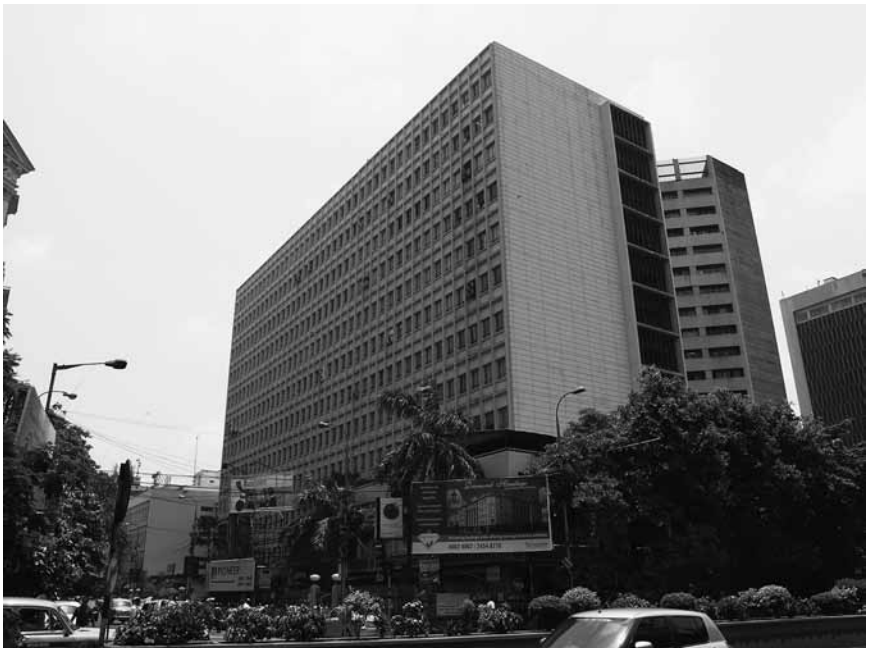
6.46 Burma Shell Building in Kolkata, 2012
