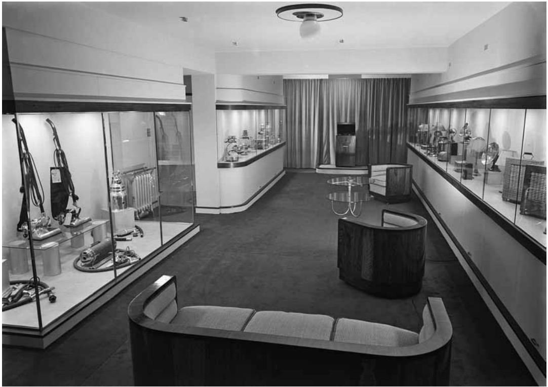
2.26 Interior of the Westminster Electric Supply Corporation Showrooms, Victoria Street, London, 1933
