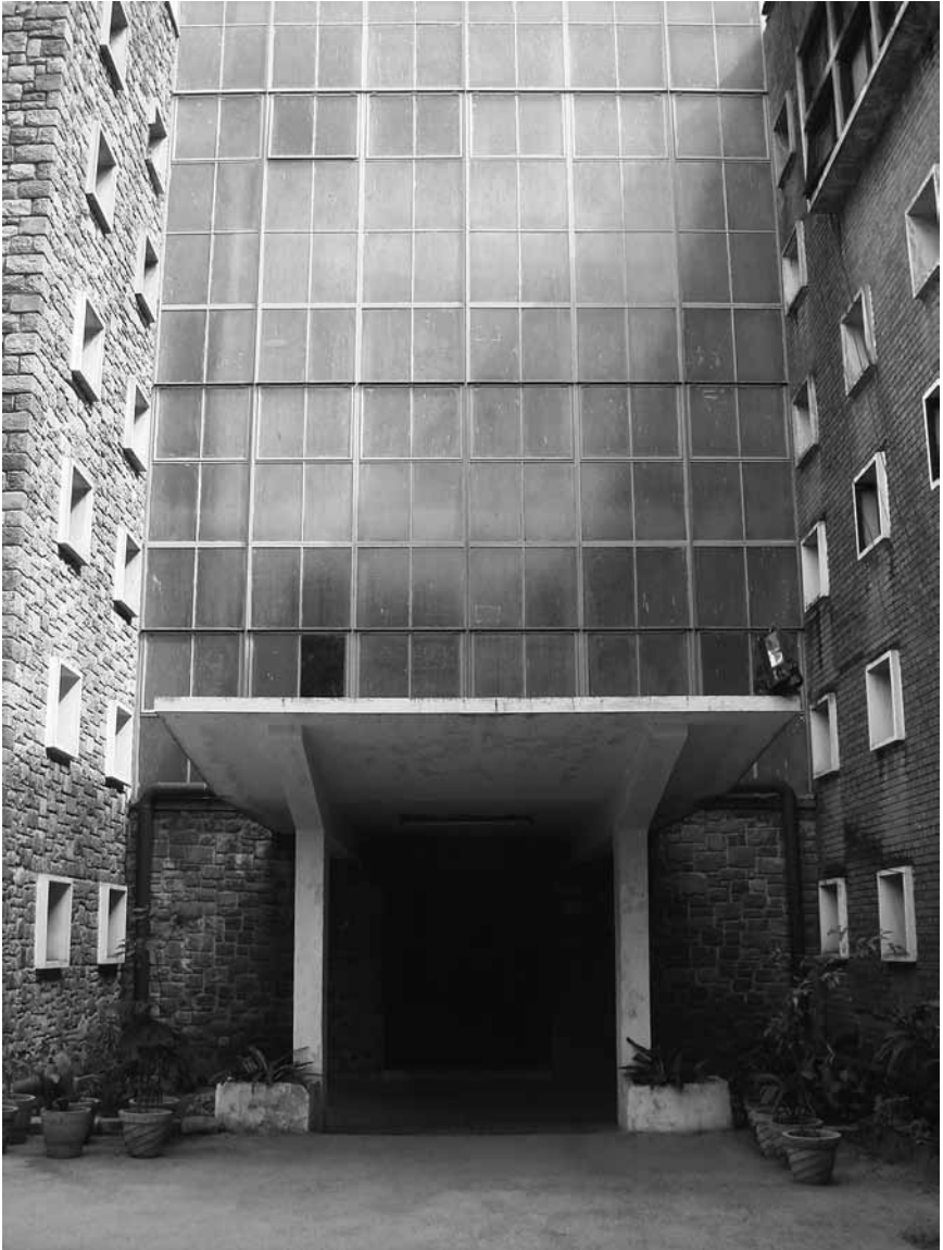
6.25 Government Press Building, entrance, 2012
