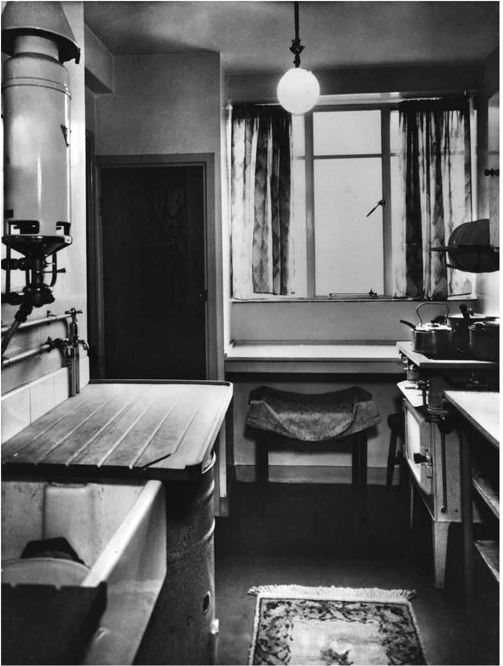
2.6 Kitchen at Kensal House, Kensington, London, 1937
