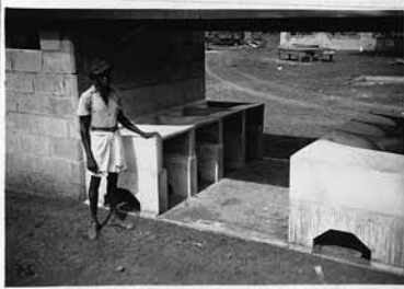
Laundry showing precast tubs with beating slab.
