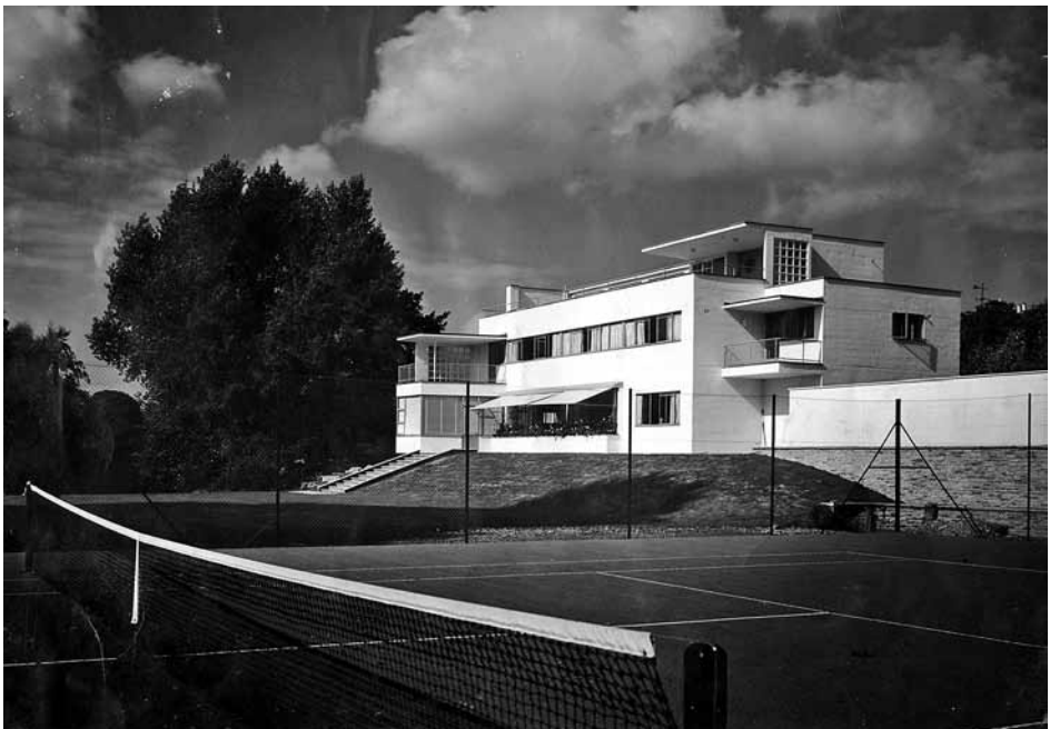
2.13 South Façade, Miramonte, Surrey, 1936
