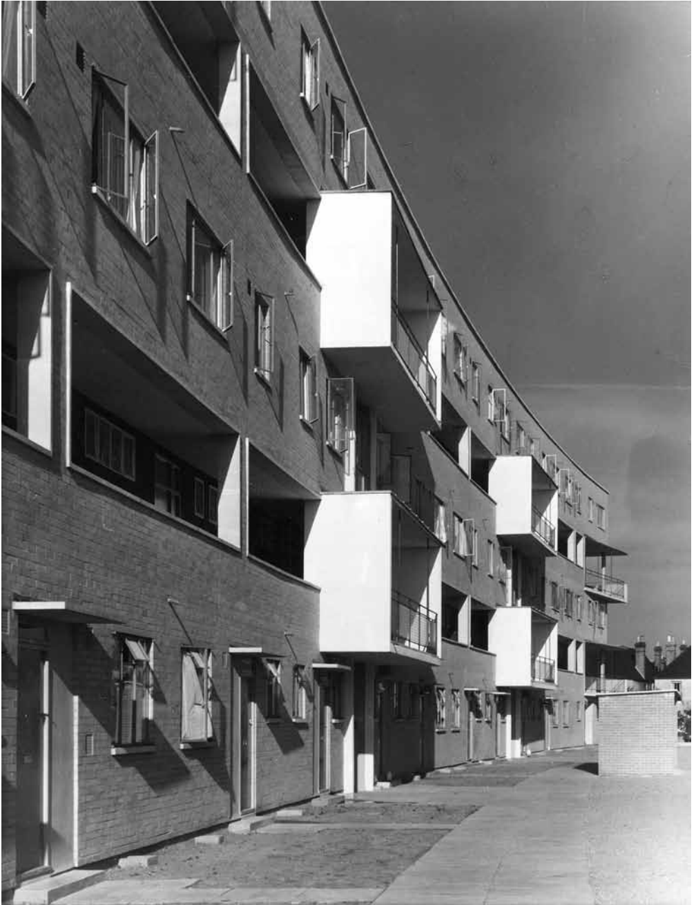
3.18 East Façade, Passfields, Bromley Road, Lewisham, London, 1951
