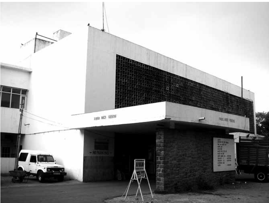
6.34 General Hospital in Sector-16, 2012
