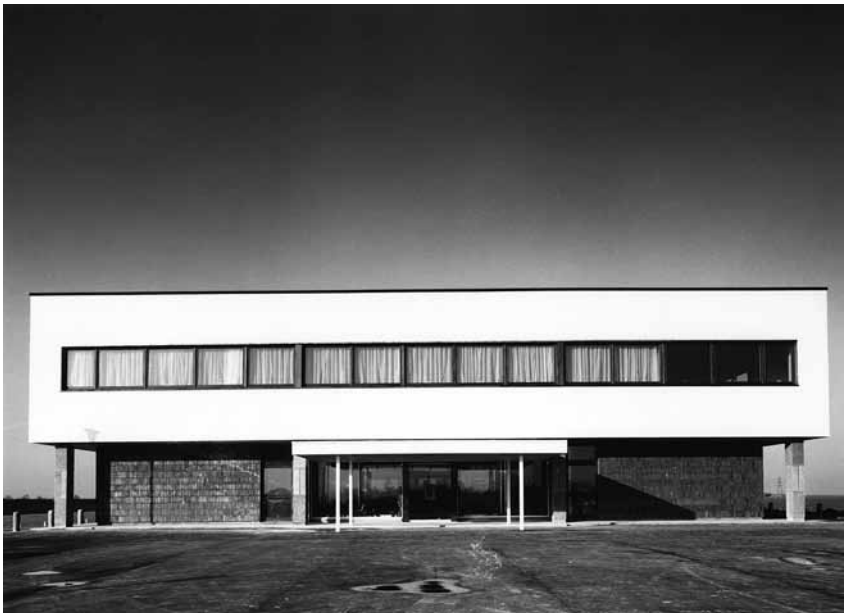
7.21 Dow Agrochemicals Office Building, King's Lynn, 1960
