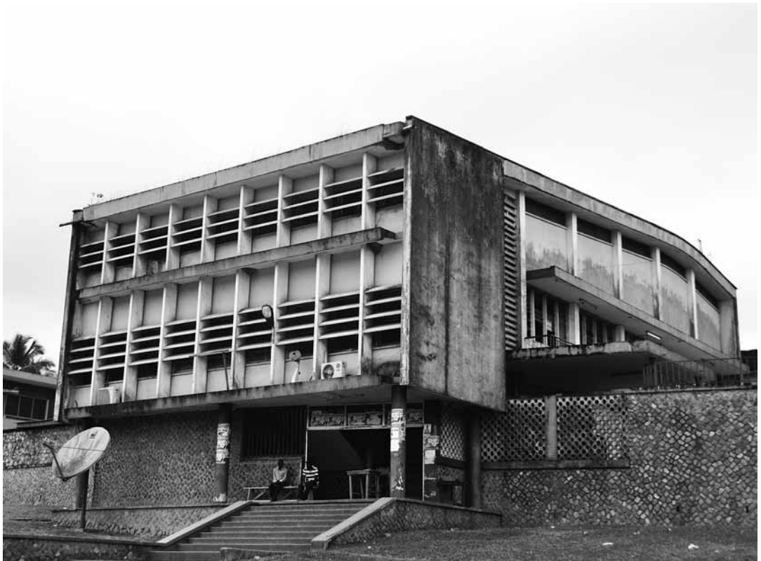
5.14 Tarkwa Community Centre, 2012
