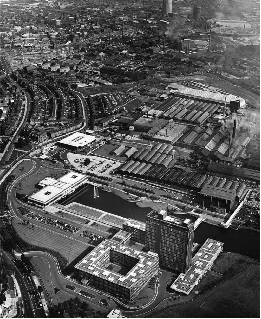
7.7 Aerial View from the West, Pilkington Brothers' Headquarters, St Helens, c. 1965
