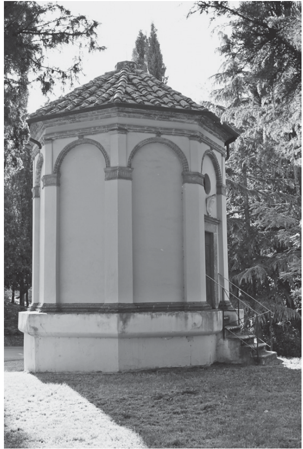
Fig. 143 Chapel of the Ascension, San Vivaldo, Montaiione, early sixteenth century (Photo: author)
