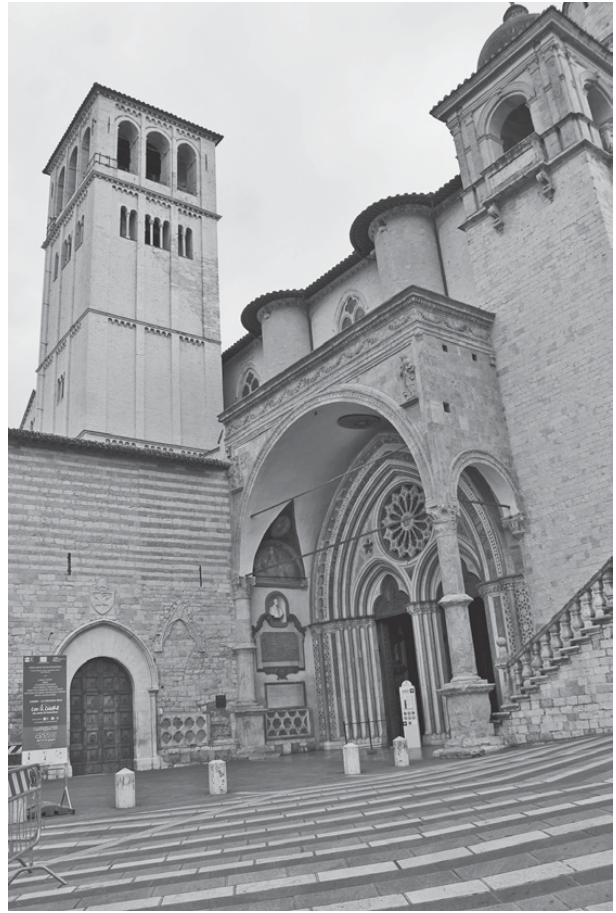
Fig. 78 Southern entrance to the Lower Church of St. Francis, Assisi (Photo: author)
