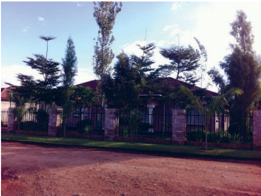
3.6 Elite housing nearing completion, Meanwood Ibex, Lusaka, June 2013.
