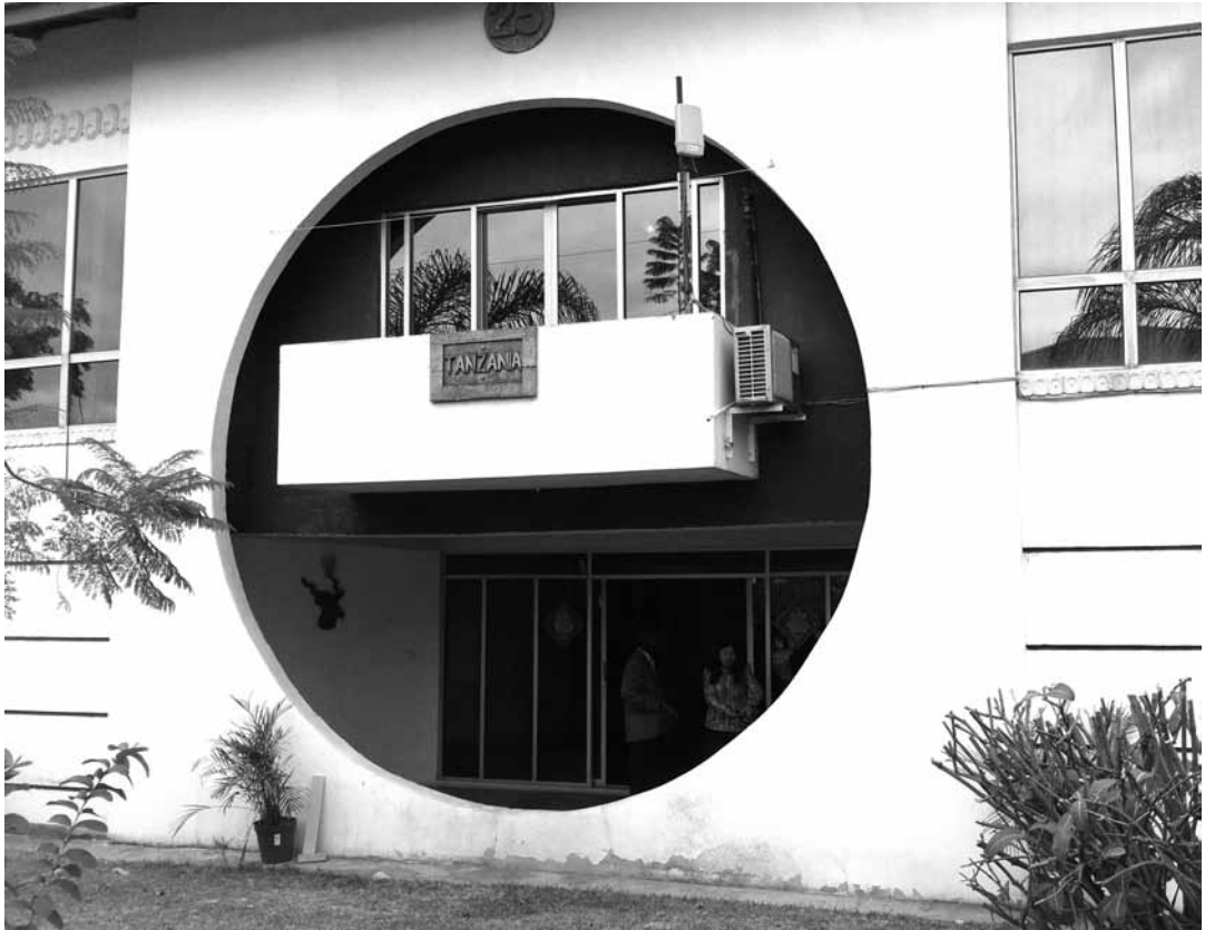
3.1 The Henan-Guoji Development Company headquarters, in Tanzania House, Millennium Village Business Park, Lusaka, June 2013. All images (3.1–3.7) courtesy of Garth Myers.
