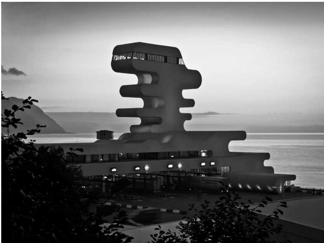
I.2 J. MAYER H. Architects, Border Checkpoint, Sarpi, Georgia. Photograph by Jesko M. Johnsson-Zahn.
