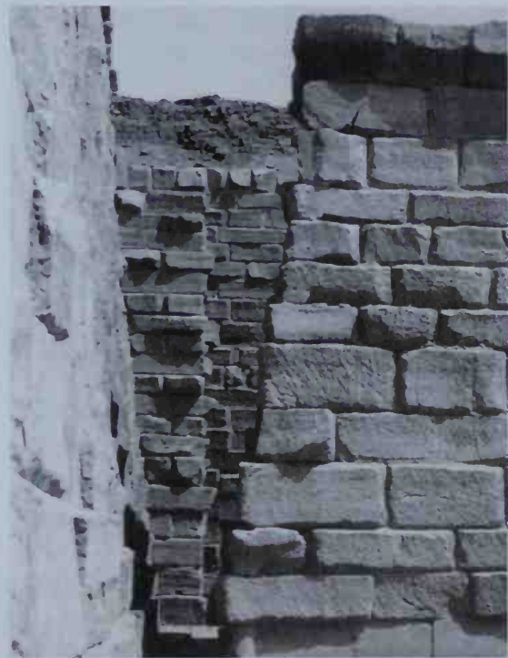
Bossed masonry at the first pylon and the barque station of Sety II at Karnak
