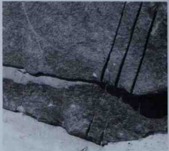
Saw marks on the basalt paving of the pyramid temple of Khufu at Giza
