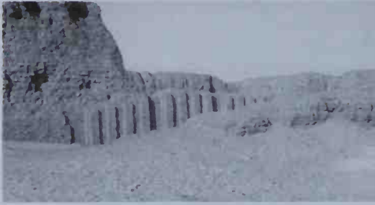
Niched enclosure wall of the funerary enclosure of Khasekhemwy at Abydos
