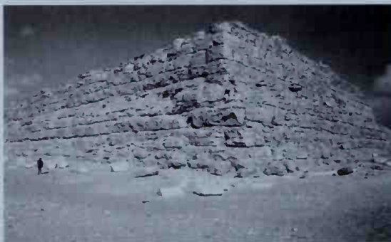
Core masonry and fallen casing blocks of the Mastabat el-Fara'un of Shepseskaf at Saqqara
