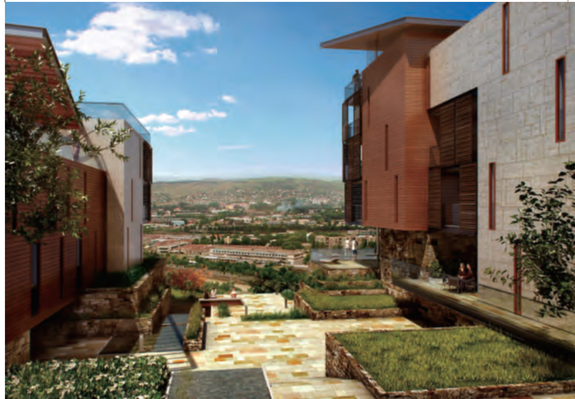
Lisi Lake's sheltered gardens are equal in scale and importance to the residences themselves.
