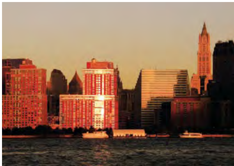
←↑ Facing west across the Hudson River at the southern tip of Manhattan, the Solaire has embedded photovoltaic panels that capture sunlight throughout the day and even at dusk, above, as it bounces off the water.
