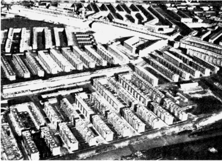
Figure 8.2: Clean-sweep planning in Europe. Slotervaart in the western suburbs of Amsterdam, from the air and on the ground
