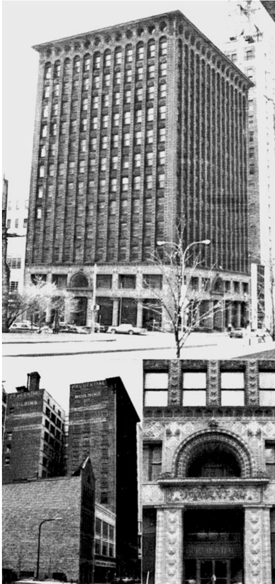
Figure 3.5: Three views of what is known to architectural historians as the Guaranty Building, Buffalo, by Adler and Sullivan, 1895, even though it has several signs declaring it to be the Prudential Building. An early skyscraper with a form which clearly reflects the steel skeleton within
