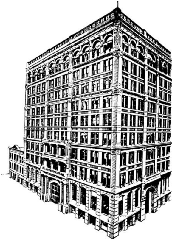
Figure 3.1: The Home Insurance Building. Designed by William le Baron Jenney, and built in Chicago in 1881, this was the first steel skeleton skyscraper, a fact disguised by the conventional decorative façade
