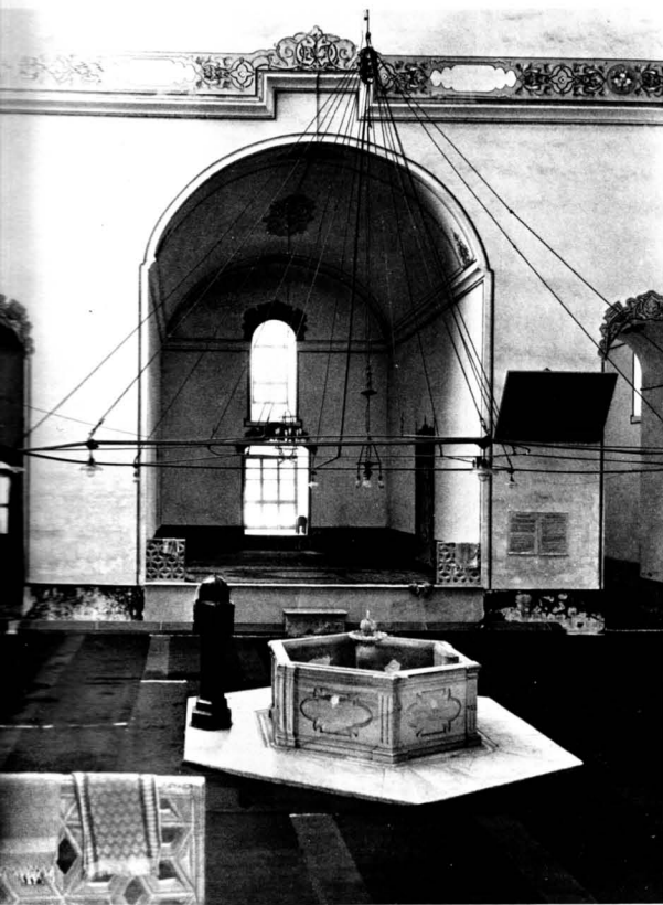
Mosque of Hüdavendigâr, Bursa 114 Interior. Side eyvan 115 Exterior
