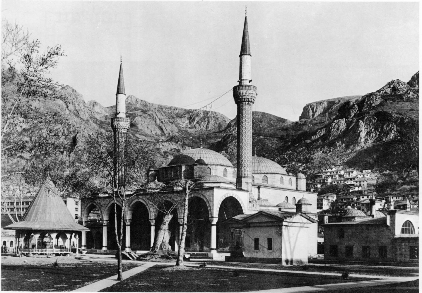
Mosque of Sultan Bayezid, Amasya 196 Exterior. Front view
