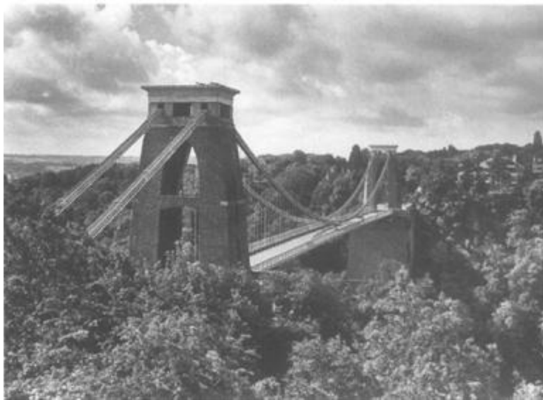
Isambard Brunei, Clifton Suspension Bridge, Bristol, 1864
