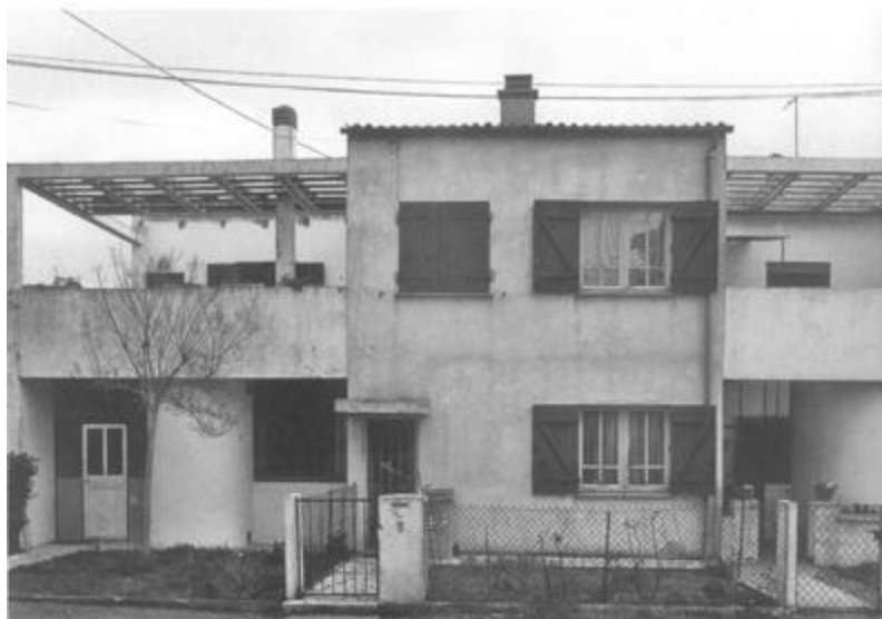
Le Corbusier, houses, Pessac, 1925 and 1995
