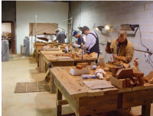
Figure 55 Winter working – preparing cut and rubbed moldings at the cutting benches. (Courtesy of Price Masonry)
