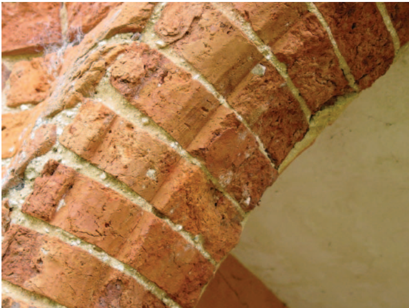
Figure 12 Green-cut moulded voussoirs to the garden gateway, Stutton Hall (Suffolk), c.1553.
