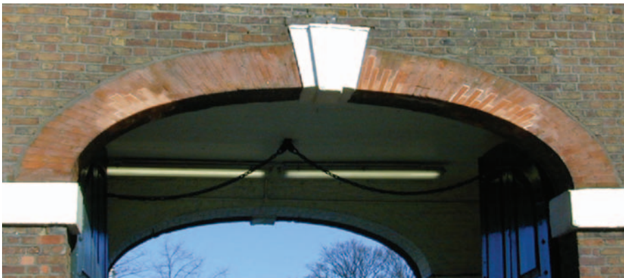
Figure 86 Semi-elliptical gauged arch to the main gateway, Chatham Dockyard (Kent), 1718. (Courtesy of Nigel A. Howard)
