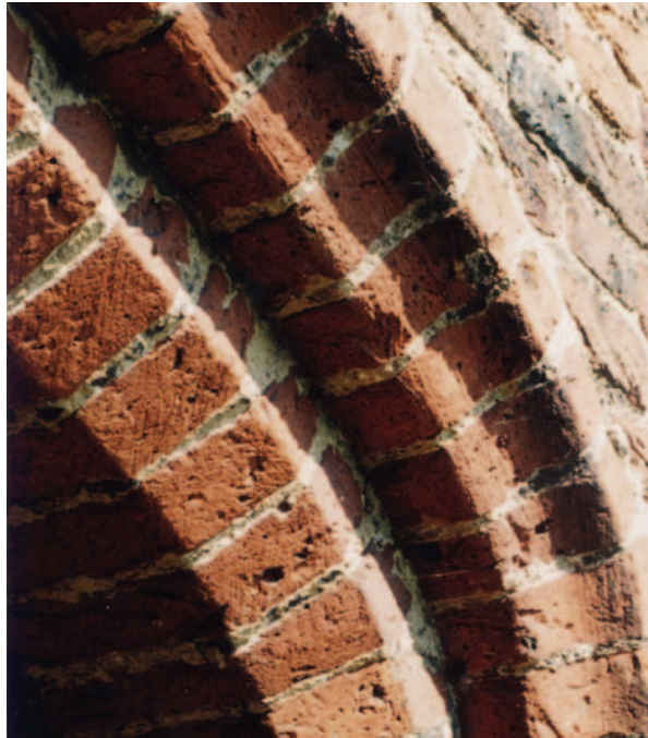
Figure 25 Cut-moulded voussoirs displaying various styled axing strokes at Kirby Muxloe Castle (Leicestershire), 1483.
