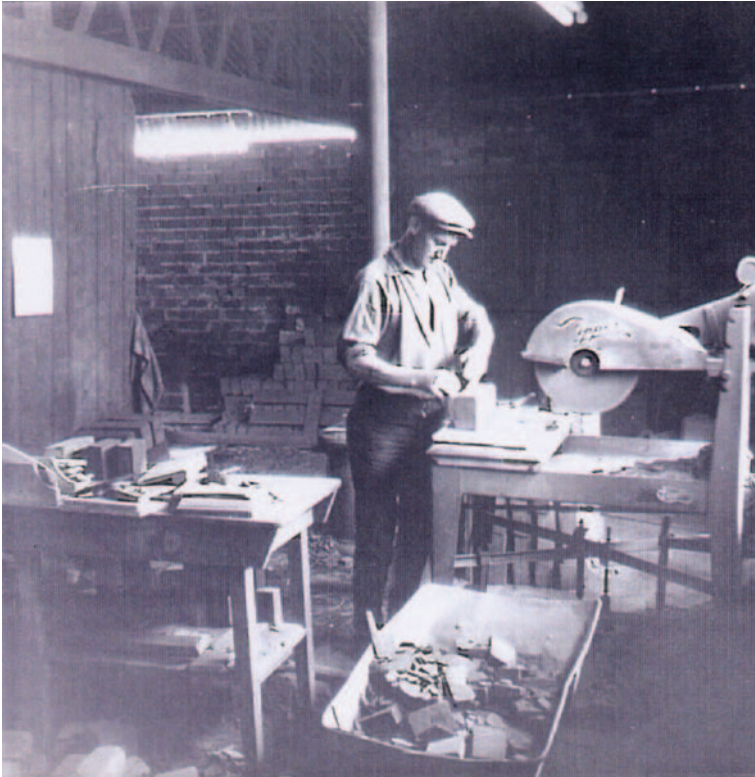
Figure 150 Cutting gauged voussoirs by bench-mounted disc-cutter at Lawrence's Warfield works (Berkshire) in the early 1950s. (Courtesy of Michael Dumbleton)
