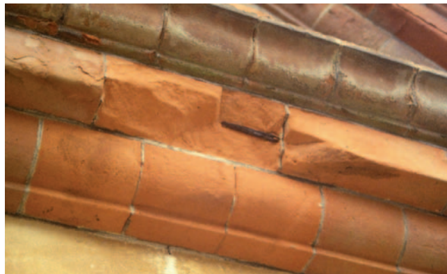
ALBERT HALL MANSIONS, KENSINGTON GORE.- Gauged brick encasement to balcony support Ironwork
