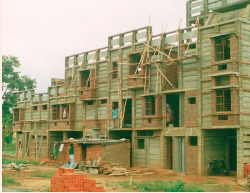
Shilpa Sindoor, Keremani Apartments, Bangalore, 1999
