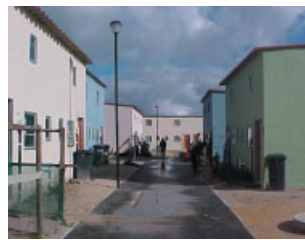
Typical interior-street configuration with pedestrian-scaled unit access.
