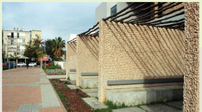
The walls in front of the centre are an element that recalls Ethiopian traditional building methods. They create semishaded spaces covered with wood twigs that mediate the ground-floor community room and the large plaza in front of it.
