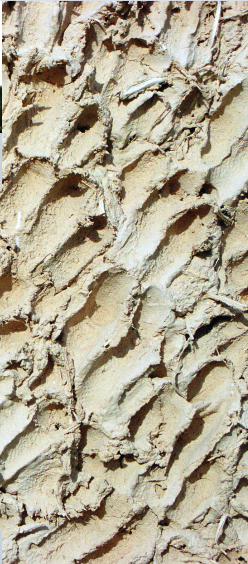
Experiments in building actual mud walls were made by the architect, but weather conditions in Israel did not permit such construction. The rich texture of the mud-like wall was achieved by hand-treating a thick layer of plaster laid over concrete masonry units.
