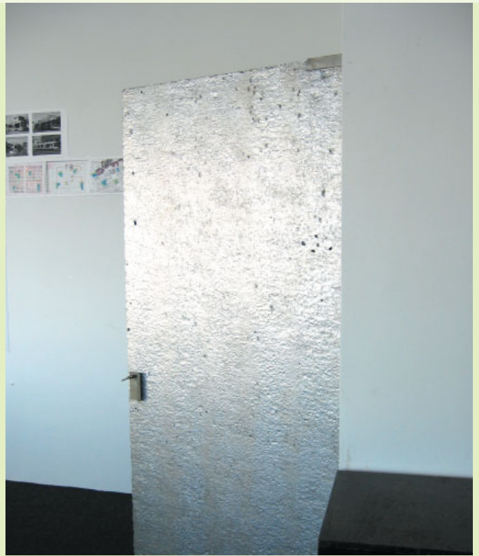
Conference Room Door, Steven Holl Architects, New York, 2000 An example of ongoing materials research: a hinged panel deriving from an aluminium insulation product.
