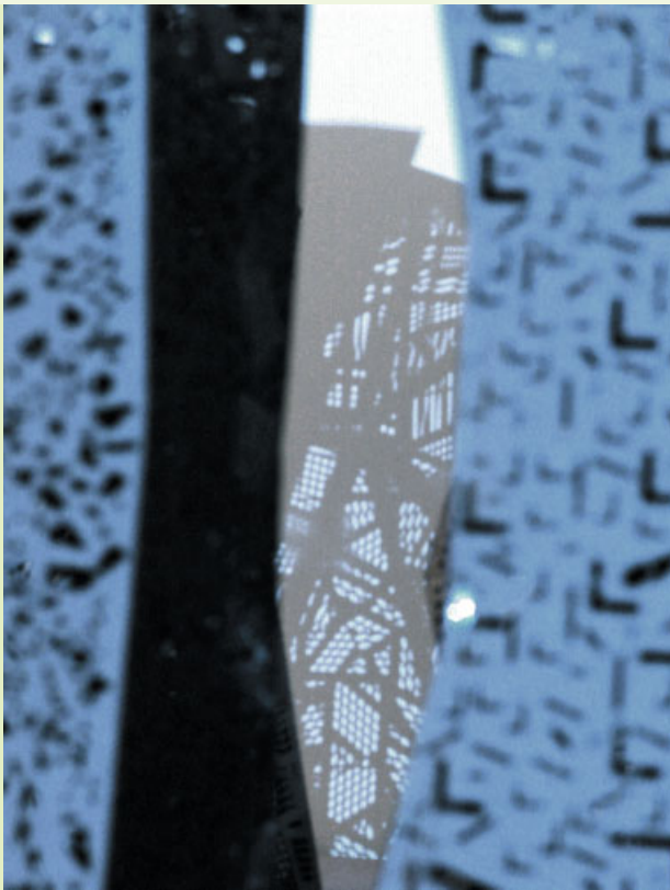
Shadow Screen, Cosmit's 'Entrez lentement' exhibit, Salone Internazionale del Mobile, Milan, Italy, 2005 Alba Flex used as porous cladding.
