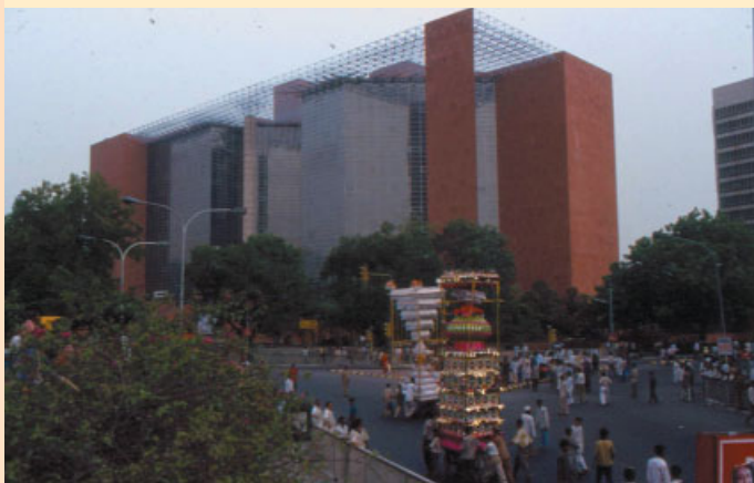
Delhi juxtapositions: a Muharram procession passes in front of Charles Correa's Life Insurance Company building.
