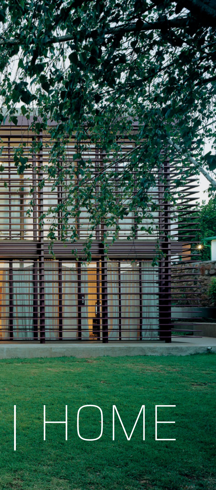
Cohen&Judin, House Gibson, Parkview, Johannesburg, 2004 The new children's (below) and parent's (above) accommodation frames the rear court against the original dwelling to the left.
