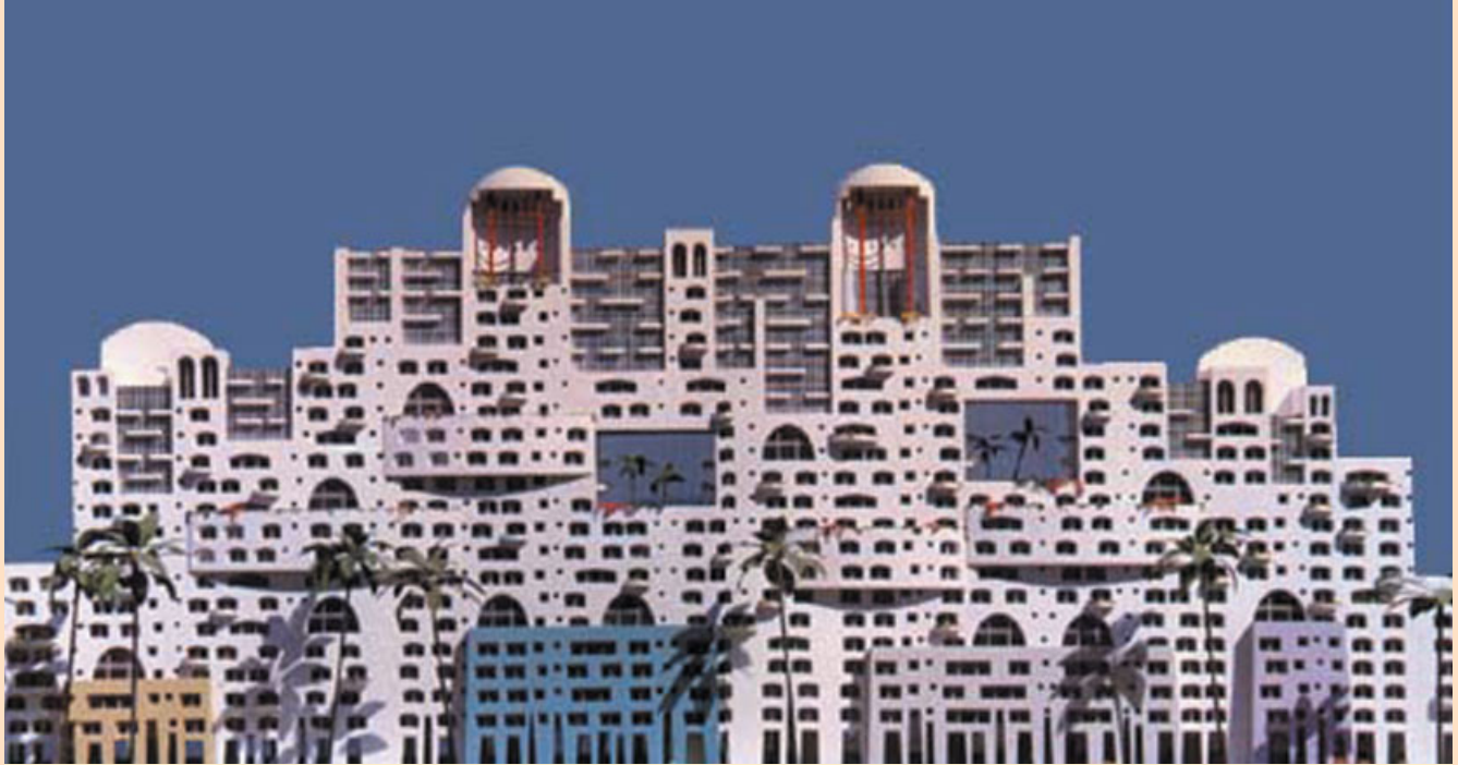
Hafeez Contractor, Lake Castle development, Powai, Mumbai, 1989 Signatures of a new living: mixed metaphors and stratospheric locations.
