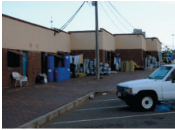
Row-attached units form a street edge with a generous trading sidewalk at Mansel Road.
