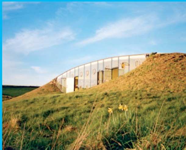
Future Systems, Marshall-Andrews House, Pembrokeshire, Wales, 1994 Fully set into the coastal landscape, this weekend retreat house has a glazed ‘eye’ that turns towards the sea.
