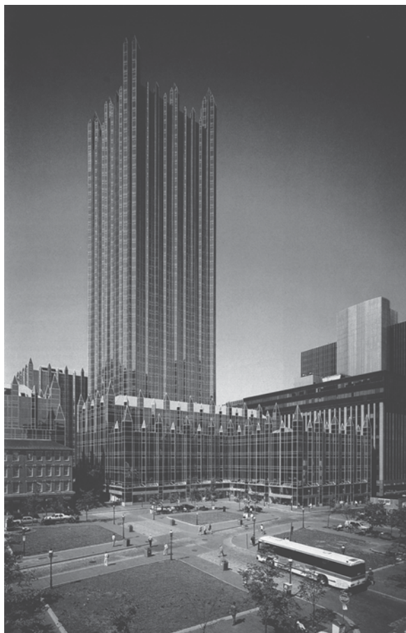
Philip Johnson and John Burgee, PPG Place, Pittsburgh, 1984. Photograph by Richard Payne, FAIA.
