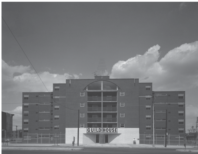
Venturi and Rauch, Guild House, Philadelphia, 1963. Photograph by William Watkins. Courtesy of Venturi, Scott Brown and Associates, Inc.
