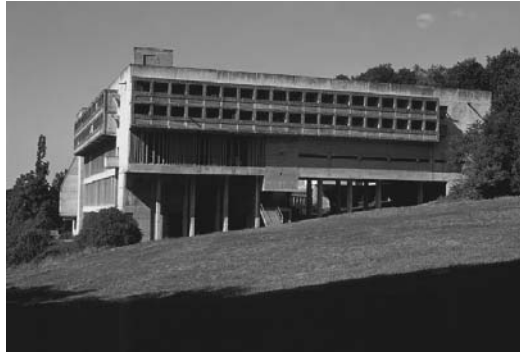
6.1 General view of Convent of La Tourette, Eveux- sur-l'Abresle, Lyons, France, 1953–1960. Architect: Le Corbusier
