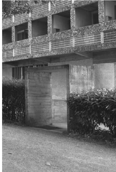
6.7 Entry portal, east side. La Tourette, 1953–1960. Architect: Le Corbusier
