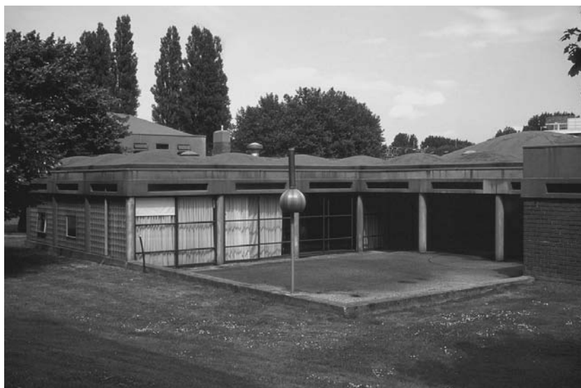
11.12 West side court. Amsterdam Orphanage, 1955–1960. Architect: Aldo van Eyck
