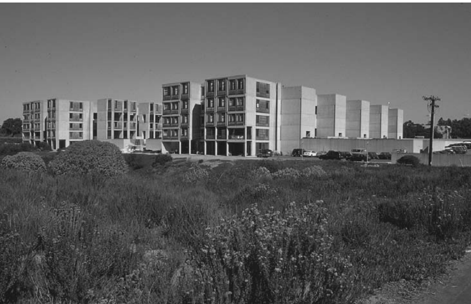
9.16 Office wing. Salk Institute for Biological Studies, La Jolla, CA, 1959–1965. Architect: Louis I. Kahn
