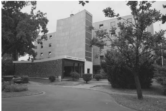
6.4 North side view of Pavillon Suisse, Paris, France, 1930–1931 Architect: Le Corbusier
