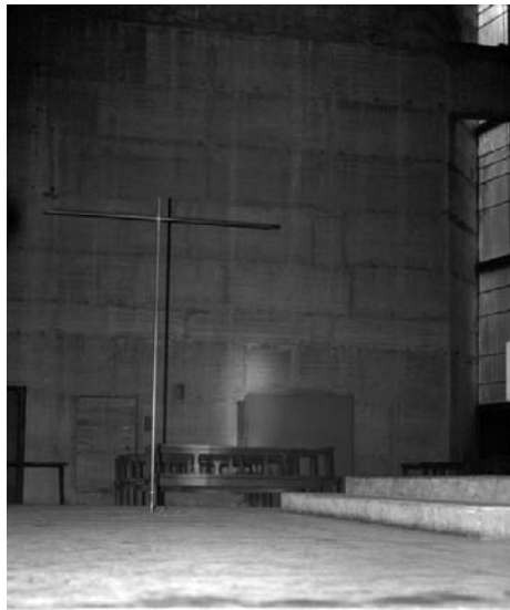
13.11 Church interior. La Tourette, 1953–1960. Architect: Le Corbusier
