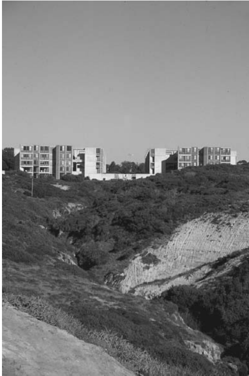
Looking east across canyon. Salk Institute for Biological Studies, La Jolla, CA, 1959–1965. Architect: Louis I. Kahn
