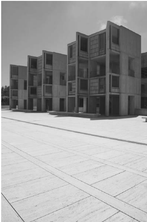
9.15 Study cells. Salk Institute for Biological Studies, La Jolla, CA, 1959–1965. Architect: Louis I. Kahn
