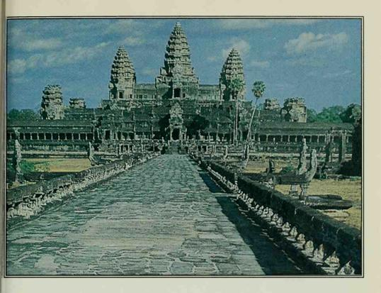
Amazingly, the vast temple was constructed without mortar and has almost no foundations, yet it remains nearly intact 1,000 years later. Only iron bars driven into stones and the temple's own weight—hold the masonry together. One striking feature of Angkor Wat is its many-tiered towers, star-shaped at their peaks.
