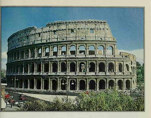
The arches of the outer wall were framed by three styles of columns: Doric on the ground floor, Ionic on the second level, and Corinthian, the most elaborate, on the third level. Eighty entrances, through arches on the ground floor, allowed for easy access.
