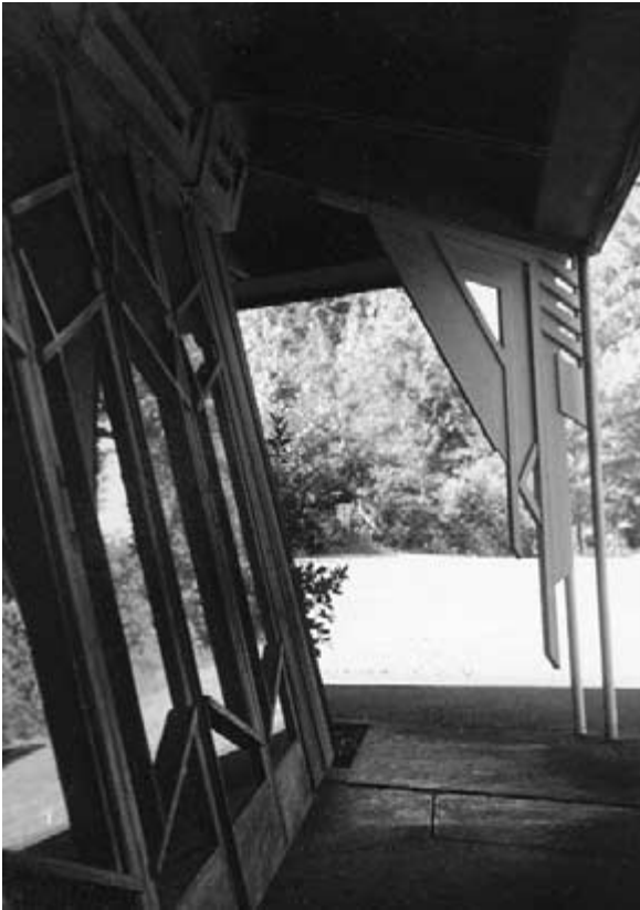
Figure 8-23 Wright designed downspouts at Auldbrass Plantation to echo the graceful draping forms of Spanish Moss. (Photograph by Charles E. Aguar. © 2002 by Berdeana Aguar.)
