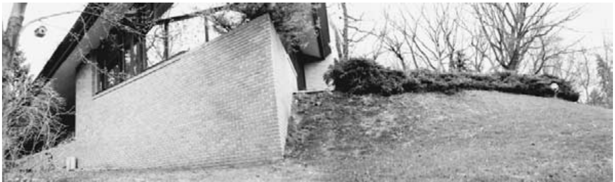
Figure 8-31 Photograph of masonry retaining base Wright conceived to address problems of irregular topography. (Photograph by Charles E. Aguar. © 2002 by Berdeana Aguar.)
