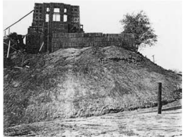
Figure 5-18 Basic mound formation of the site for the Charles W. Ennis House (1923–1926) in Hollywood, California. (Courtesy of Eric Lloyd Wright.)
