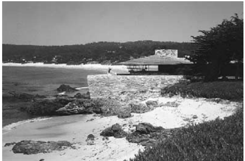
Figure 8-32 Masonry retaining base of terrace for Della Walker House (1948–1952) in Carmel, California. (Photograph by Charles E. Aguar. © 2002 by Berdeana Aguar.)
