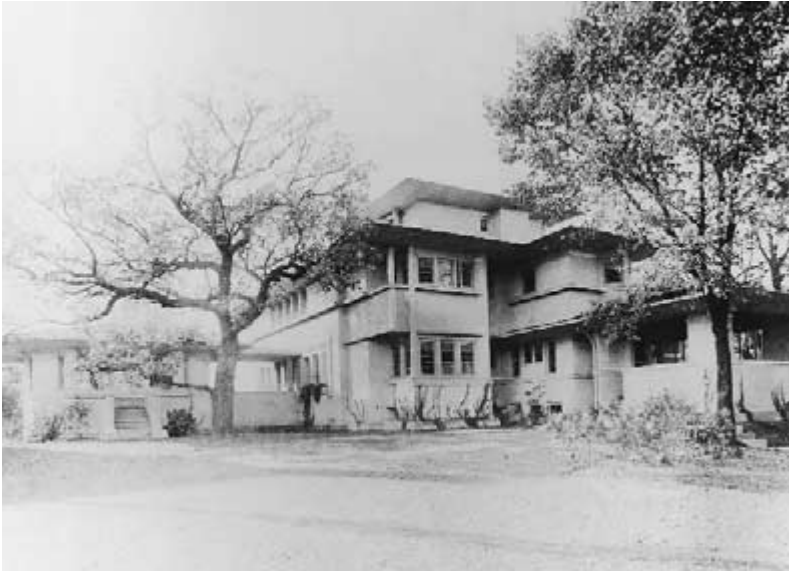
Figure 3-17 Historic photograph shows the Fricke garden pavilion and specimen Oak that inspired zero-lot-line siting. ( Out-of-copyright photograph of record from Wasmuth Portfolio, 1911. )
