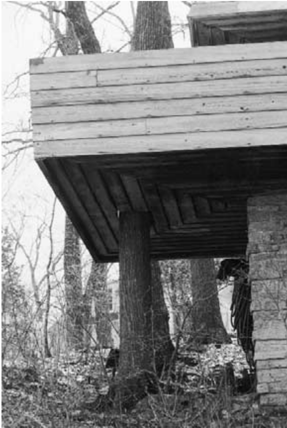
Figure 8-17 Photograph shows linden tree protruding through Pew deck. Wright originally planned to save two trees. (Photograph by Charles E. Aguar. © 2002 by Berdeana Aguar.)
