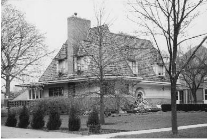
Figure 2-15 Appearance of the Williams House after the earthen terrace was leveled and plantings were allowed to obscure Wright's design intent. (1993 photograph by Charles E. Aguar. © 2002 by Berdeana Aguar.)
