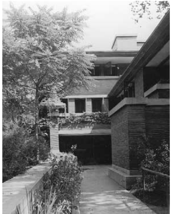
Figure 3-76 Entrance court and entry garden approach to Robie House. (Photograph by Gilman Lane. Courtesy of Gilmore Collection, Oak Park Public Library, Oak Park, Illinois.)
