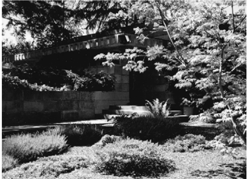
Figure 8-61 The Tracy House appears to nestle into its site. (Photograph by Charles E. Aguar. © 2002 by Berdeana Aguar.)
