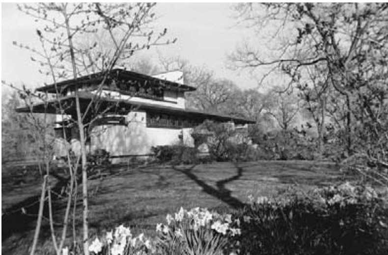
Figure 3-54 A photograph of the Ferdinand F. Tomek House (1904–1905) in Riverside, Illinois, shows cantilevered extension of roofline. (Courtesy of Maya Moran Manny.)
