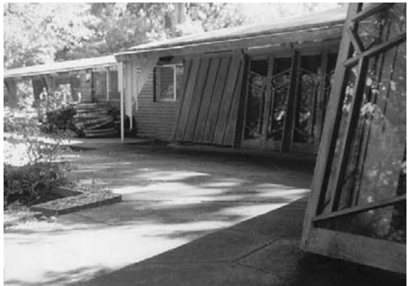
Figure 8-22 At Auldbrass Plantation, Wright battered walls of Native Cypress at a 9-degree angle to harmonize with sloping trunks of Live Oak trees. (Photograph by Charles E. Aguar. © 2002 by Berdeana Aguar.)
