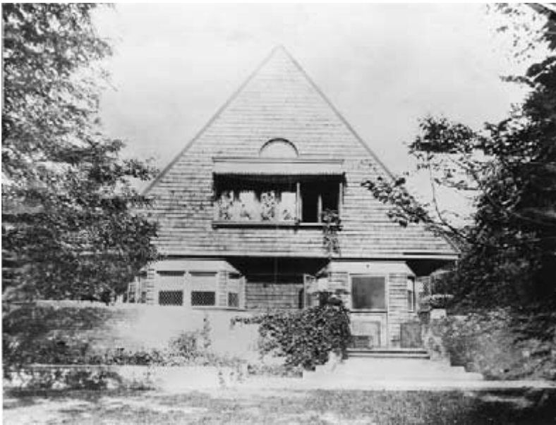
Figure 2-2 West facade of Frank Lloyd Wright’s original shingle-style Home (1889) in Oak Park, Illinois. (Courtesy of The Frank Lloyd Wright Preservation Trust, Oak Park, Illinois.)
