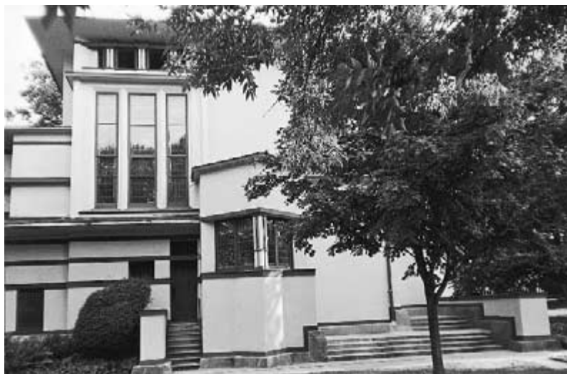
Figure 3-15 A photograph of the 1901 William G. Fricke House in Oak Park, Illinois, depicts the effect of zero-lot-line siting. (1992 photograph by Charles E. Aguár. © 2002 by Berdeana Aguár.)
