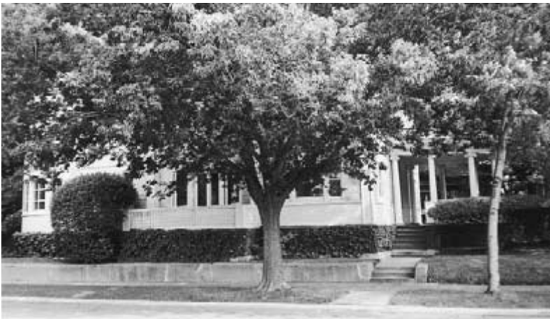
Figure 2-9 Low retaining wall and masonry water table visually minimize vertical mass of Blossom House. (Photograph by Charles E. Aguar. © 2002 by Berdeana Aguar.)
