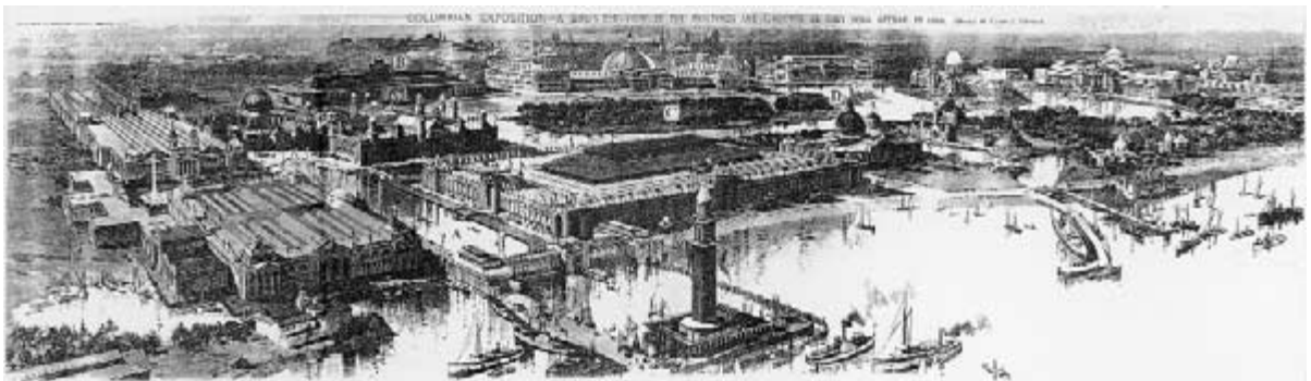
Figure 1-4 Bird's-eye perspective of buildings and grounds, World's Columbian Exposition, Chicago, Illinois. ( Supplement to Harper's Weekly, December 19, 1891. )
