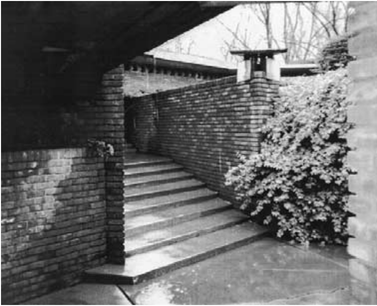
Figure 8-50 Rotation of Palmer House necessitated adding 12 entry steps. (Photograph by Charles E. Aguar. © 2002 by Berdeana Aguar.)
