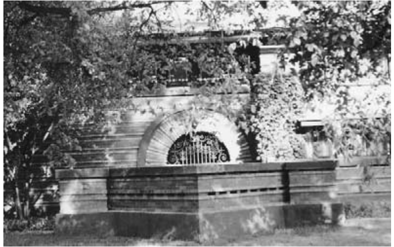
Figure 3-24 The prow of the Heurtley terrace provides privacy and shields the main entry from prevailing winter winds. (Photograph by Charles E. Aguar. © 2002 by Berdeana Aguar.)
