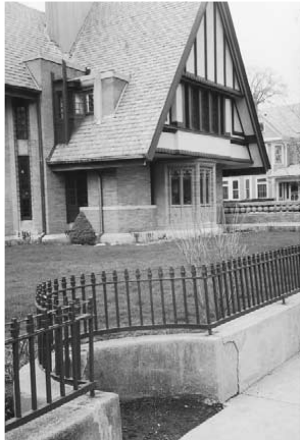
Figure 2-18 The Moore House's ornamental wall-fence was arced to accommodate the trunk of an existing tree (since removed). (Photograph by Charles E. Aguar. © 2002 by Berdeana Aguar.)
