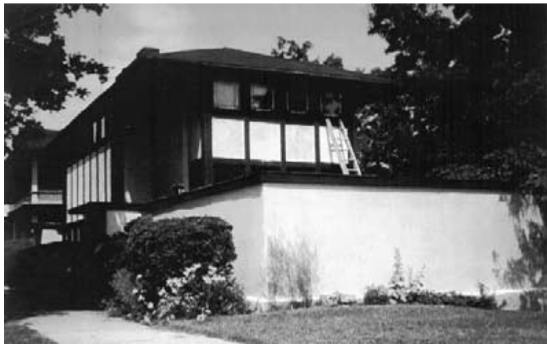
Figure 3-52 A 1992 photograph shows the proximity of the Hardy House to Racine’s Main Street, just to left of sidewalk. (Photograph by Charles E. Aguar. © 2002 by Berdeana Aguar.)
