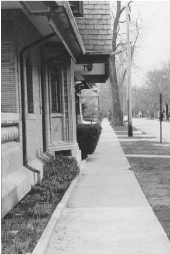
Figure 2-17 The north facade of the Moore House encroaches on the public right-of-way along Superior Street. (Photograph by Charles E. Aguar. © 2002 by Berdeana Aguar.)
