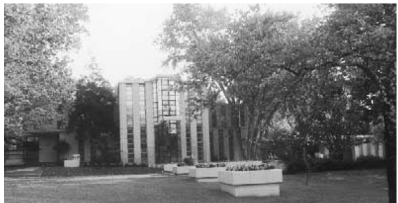
Figure 6-9 A unique rhythmic detail of Westhope’s exterior walls featured alternating floor-to-ceiling columns of concrete blocks and windows. (Photograph by Charles E. Aguilar. © 2002 by Berdeana Aguilar.)
