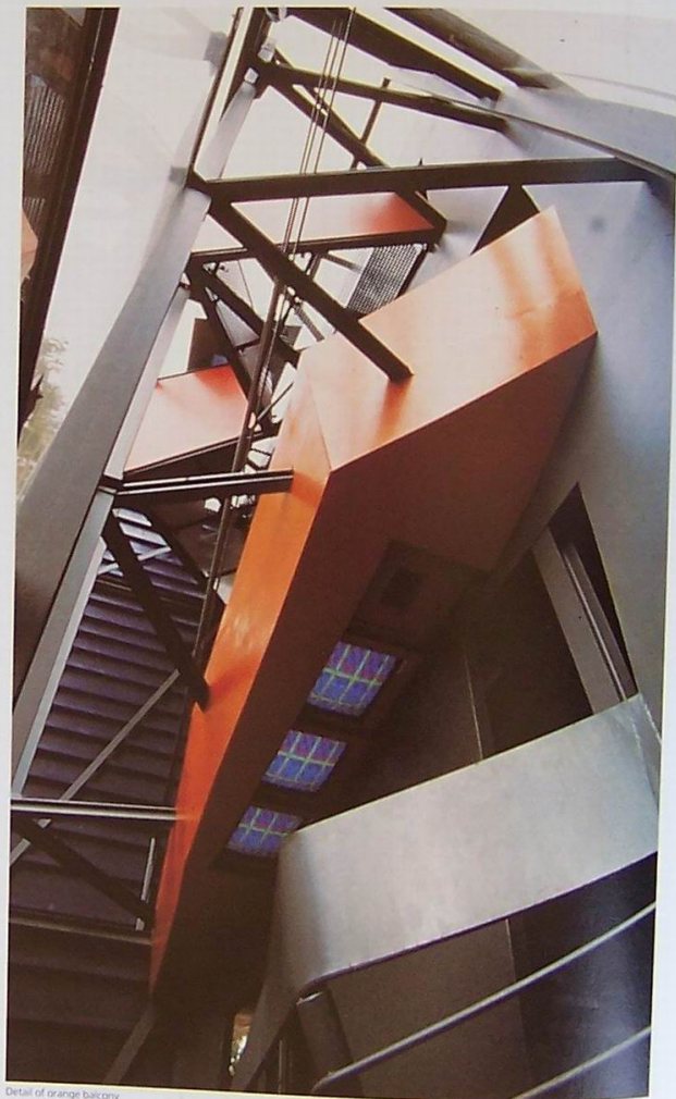
Detail of orange balcony
