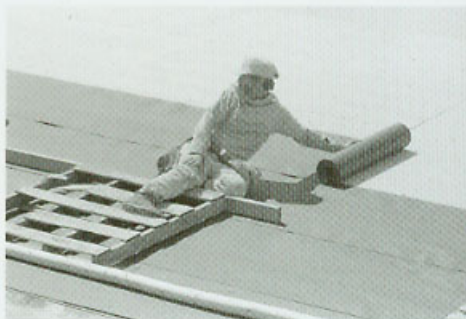
Covering a new roof with waterproof membrane
