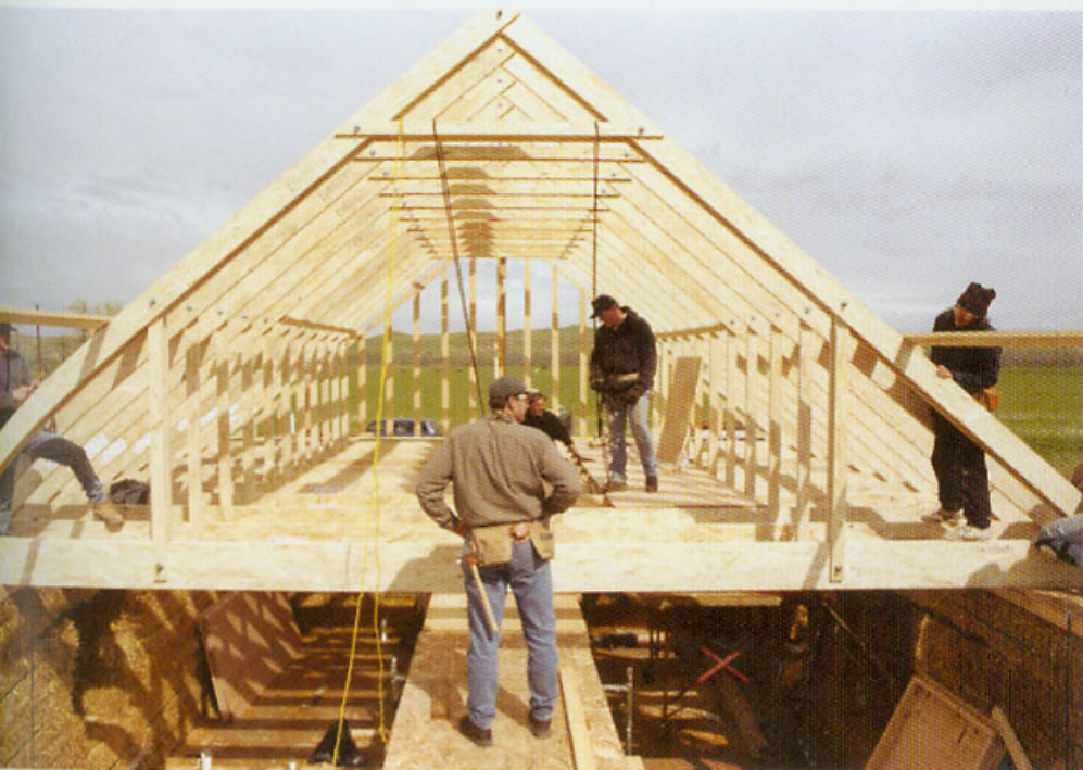
Steep roofs require more material and are harder to work on, but the tradeoff is loft space.
