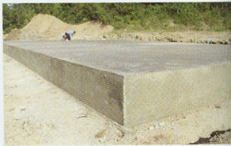
The completed slab awaits straw bales.
