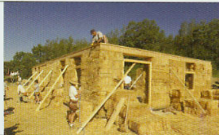
Left and right: Extra bales come in handy for temporary stairs and scaffolding.
