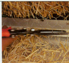
Trimming lath within the weep screed
