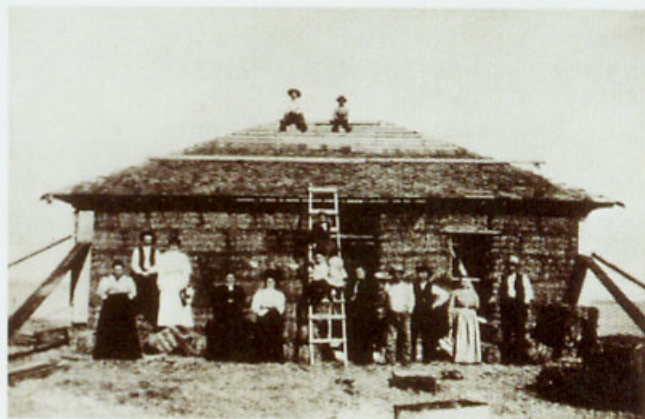
The Simonton Family Home, Purdum, Nebraska, built c. 1908: An early example of a load-bearing bale building that is said to have been constructed with prairie hay cut after a frost.
