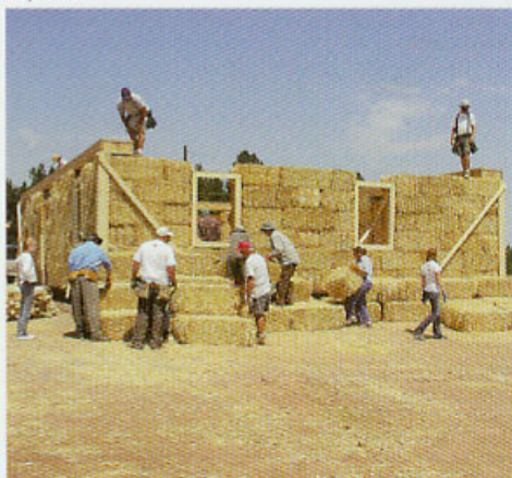
Build straw bale scaffolding along walls where RBA sections will be placed.
