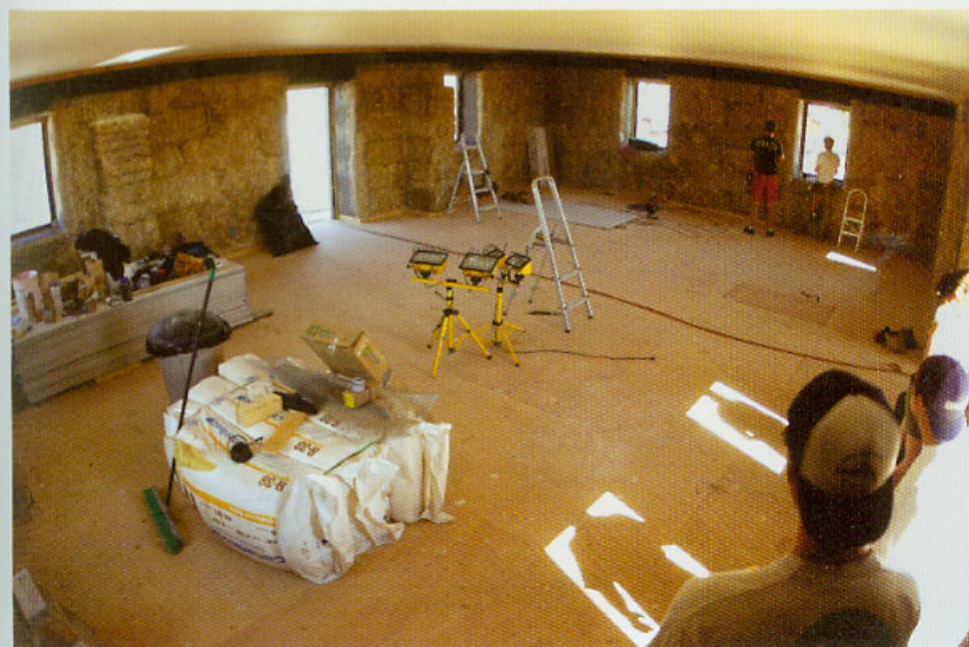
Install ceiling drywall before starting stucco work to help compress the bale walls.
