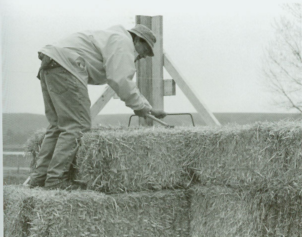
Bent rebar staples connect bales at the corners.
