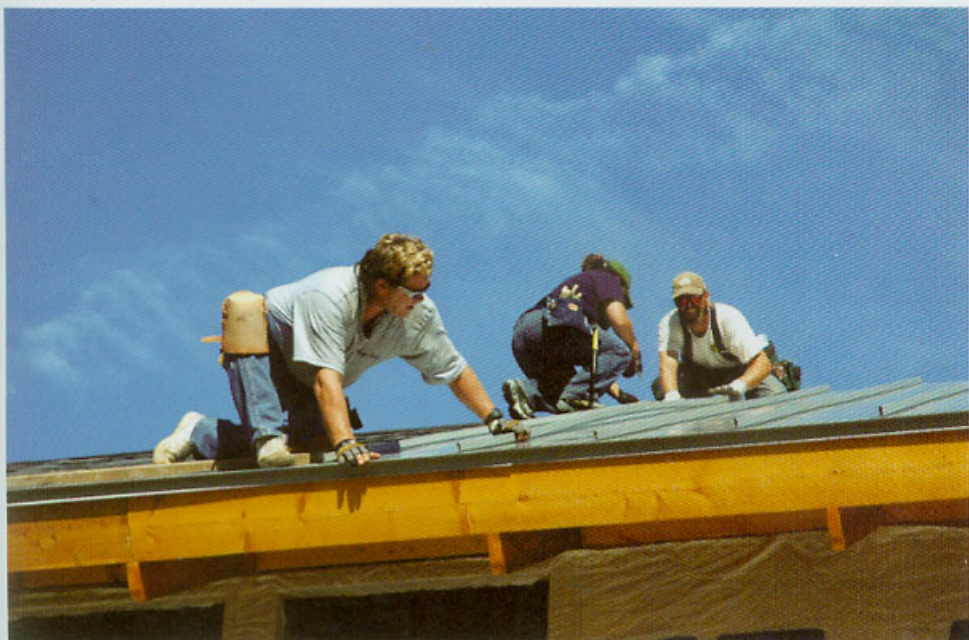
A metal roof protects bale walls for years to come.
