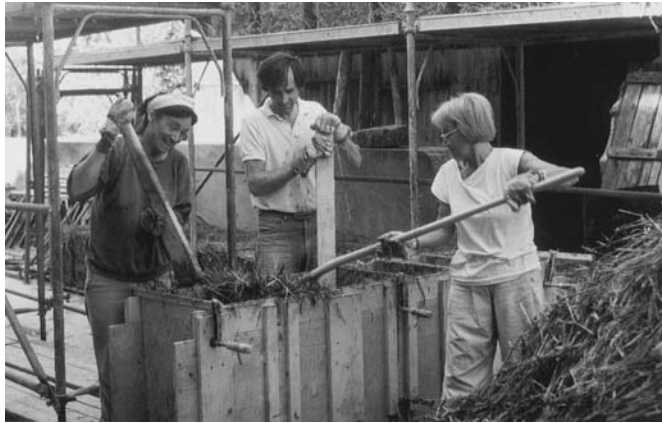
7.1 Making light-weight straw loam blocks
