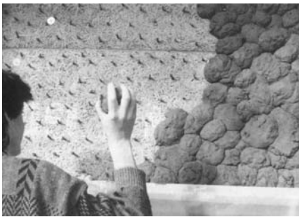
11.5 Spraying light-weight loam plaster 11.6 Lightweight loam plaster with expanded clay (1–4 mm) 11.7 to 11.8 Thrown plaster in a winter garden
