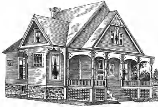
spindlework on porch
