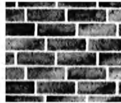
raking stretcher bond
