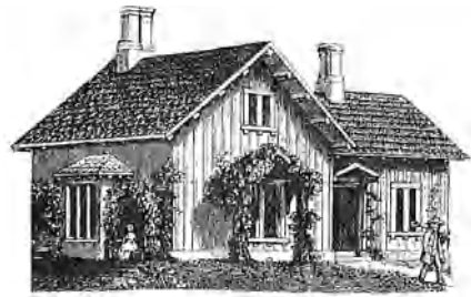
cottage with bracketed eaves
