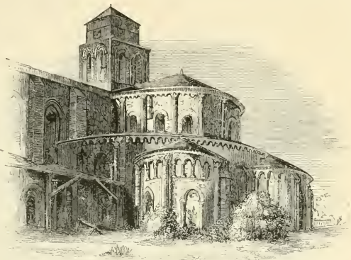
506. View of Chevet at Fontevrault. From Faultrier.
