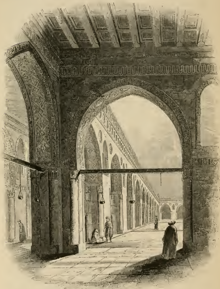
315. Mosque of Ebn Touloun at Cairo. From Coste's Architecture Arabe .
