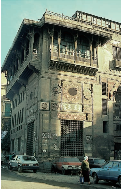
ABOVE: The sabil-kuttab of Qa'it Bay.
