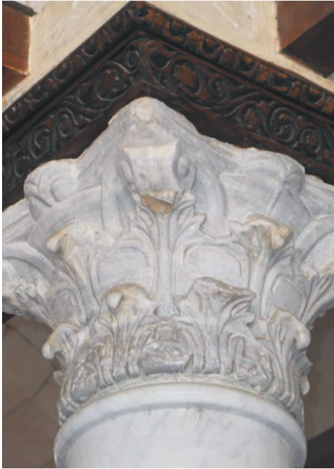
ABOVE: Mosque of Amr ibn al As: Decorated architrave with stump of broken tie-beam.
