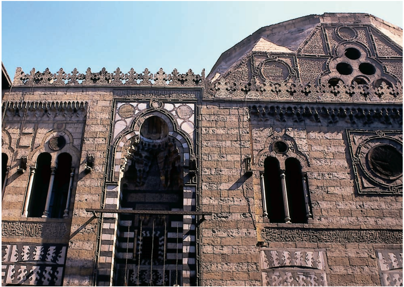
ABOVE: The mausoleum and khanqah of Sultan al-Ghuri.
