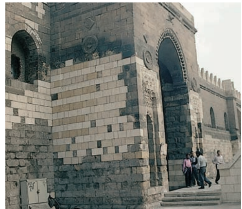
ABOVE: Mosque of Sultan al-Zahir Baibars.
