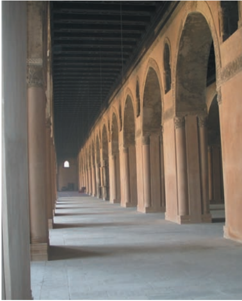
ABOVE: Piers in the prayer hall of Ibn Tulun's mosque.
