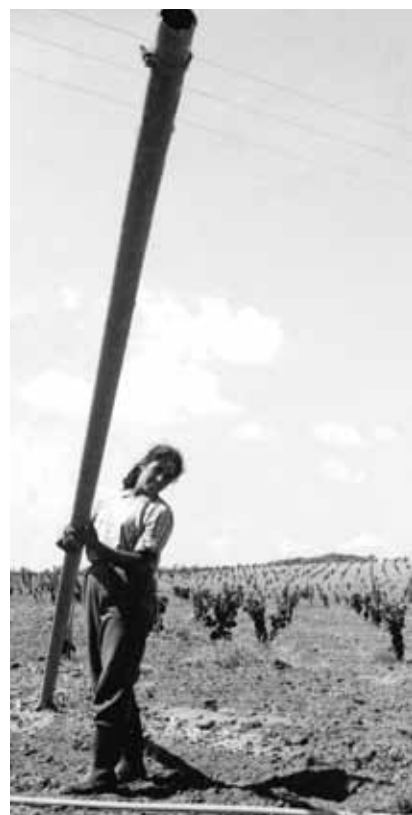
An early Jewish settler laying water pipes to irrigate the newly planted trees on a kibbutz near Ashkelem in Israel, mid-20th century.
