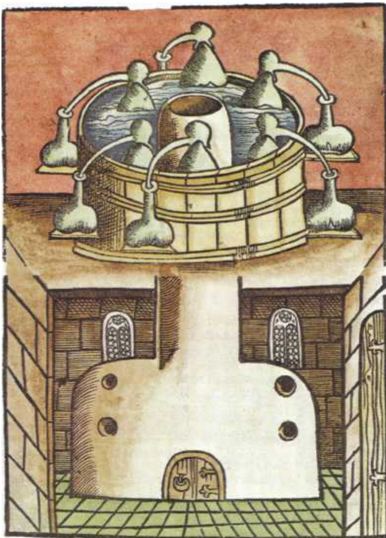
Left: the alchemist's water bath or bain-marie , a woodcut of 1519. The substances in the glass vessels suspended in the water were warmed only gradually by the furnace below the bath.
