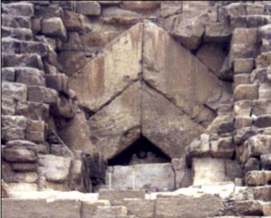
Gigantic blocks in Chephren pyramid weigh over 70 tons each and are many stories above ground.
