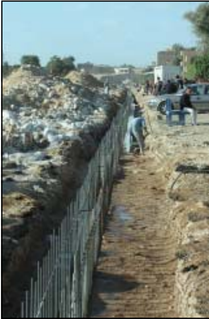
Early construction phase
