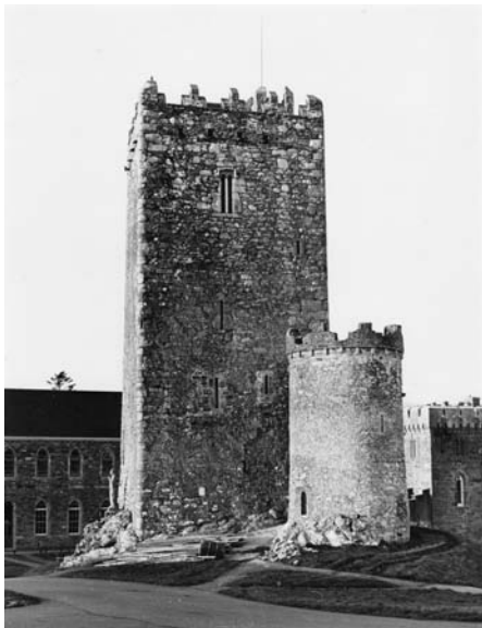
Drishane Castle, Co. Cork. © Department of the Environment, Heritage and Local Government, Dublin.
