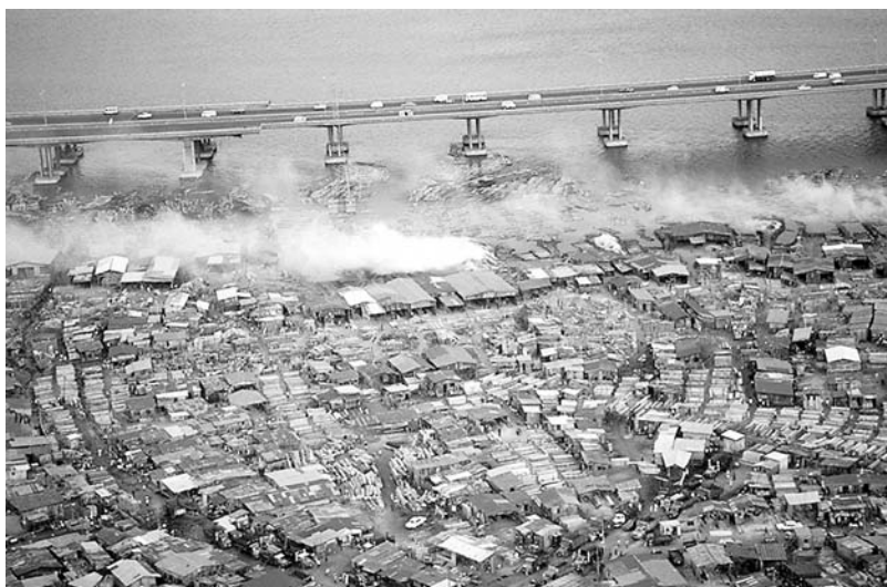
FIGURE 13. Lagos 2000. Highway bridge and a world of small-scale production and commerce. Source: Edgar Cleijne; used by permission.
