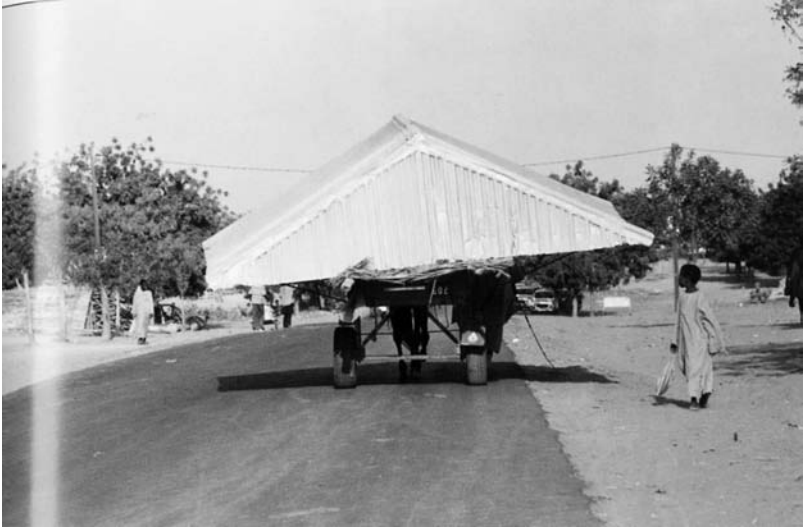
FIGURE 15. Roof delivery: how Touba is being constructed. Source: Dr. Cheikh Guèye; used by permission.
