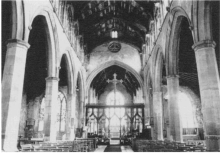
Figure 5.1 The parish church of Gedney, Lincolnshire, looking from west to east. This fully developed church dates predominantly to the thirteenth and fourteenth centuries. It consists of a structurally distinct chancel and nave, and aisles (with their own altars) to the north and south of the nave, divided from the nave by large arcades that would have been screened. The screen below the chancel arch is a nineteenth-century reconstruction of the medieval arrangement.
