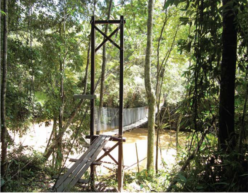
Plate 11. The completed Apir Long Da'an suspension bridge. Source: Photograph by Ian Ewart.
