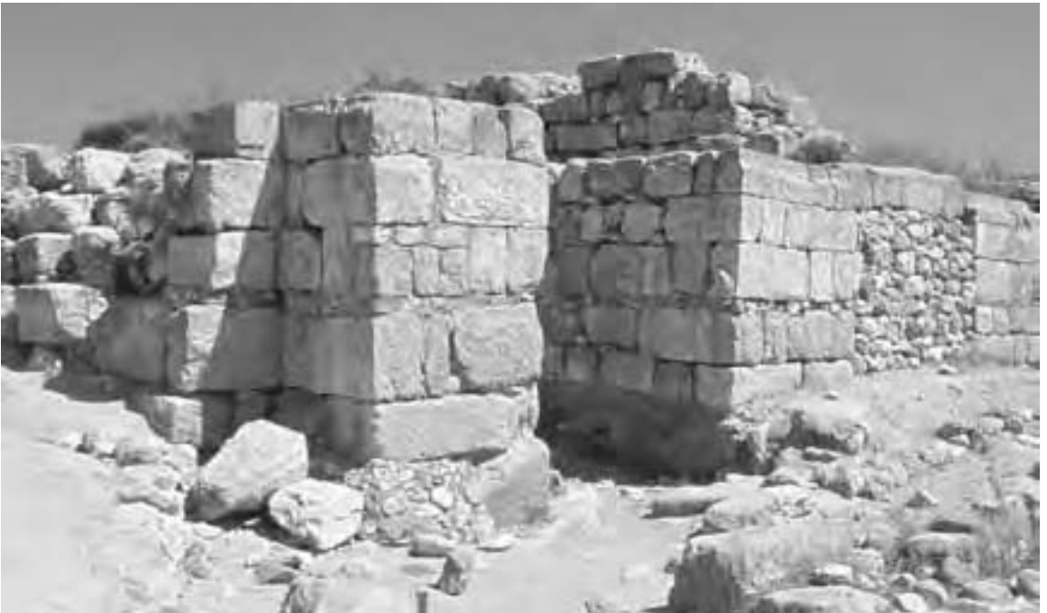
9.10a (above) Iron 2 city gate at Hazor. 9.10b (below) Iron 2 city gate at Megiddo (Photos courtesy of Zev Radovan, Land of the Bible Picture Archive)
