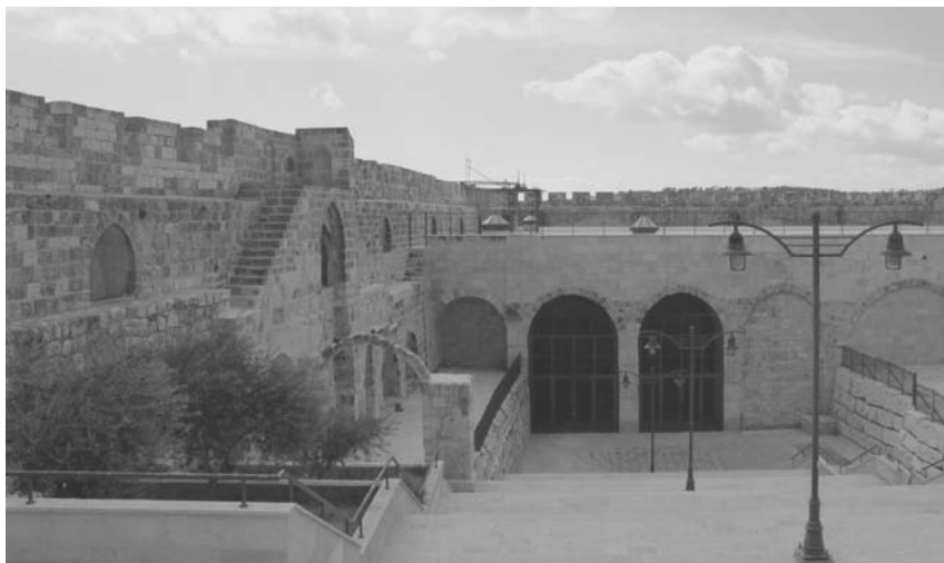
5.4. Recent restoration of the inside of the southeast corner of the temple mount, near the Triple Gate.
