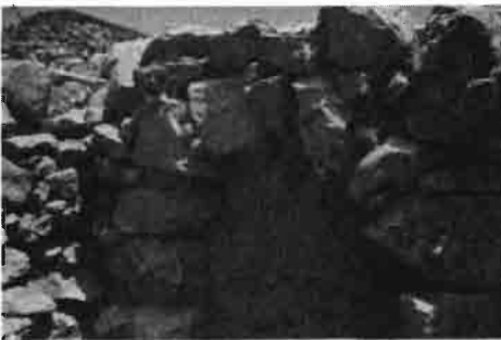
An arch with keystone from what was probably the stable of a house at Ai. From the eighth century B.C., it is one of the earliest such structures found in Israel.
