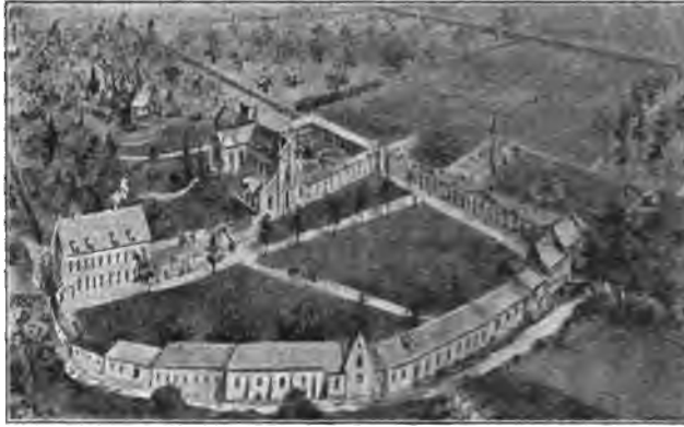
ABBAY OF TONGERLOO, BELGIUM
