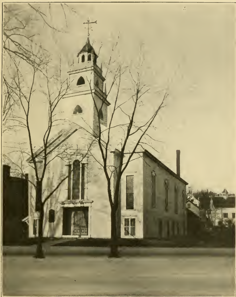
THE CONGREGATIONAL CHURCH AT TILTON, NEW HAMPSHIRE
