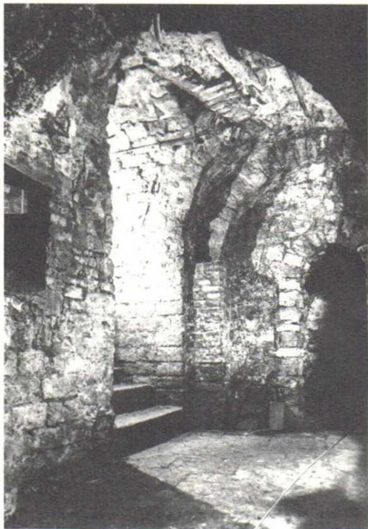
Fig. 50. Washing well, the Mikve , next to the Worms synagogue. The MaHa-RIL, and other Jews, would have used the well for washing before going to the synagogue. The well is still much as it was in the 14th century. The nearby synagogue has been rebuilt since WWII. Editor's photograph, 1990.
