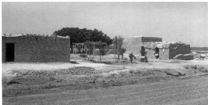
Plate 1b: Permanent Buildings with Tent Roof (Syria).
