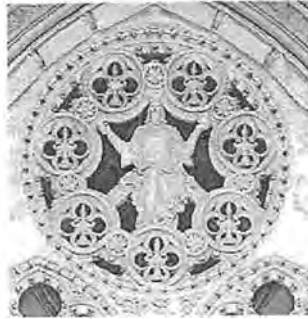
Lesser Rose Window of the Cathedral of St. John the Divine in New York City, world's largest cathedral (and still being built). Note its heptagonal design, one of the very few sevenfold Rose Windows in existence.
