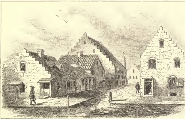
CORNER OF BROAD STREET AND EXCHANGE PLACE
