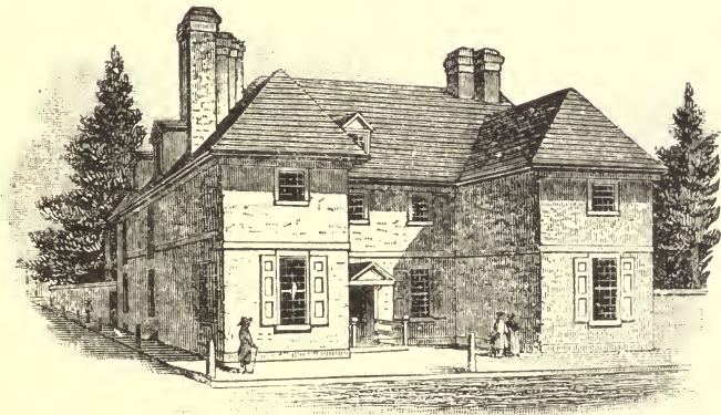
THE "SLATE-ROOF HOUSE"
