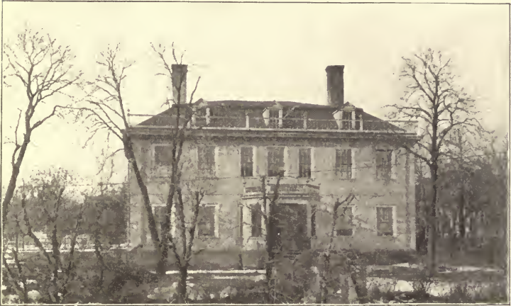
THE SCHUYLER MANSION, ERECTED IN 1761
