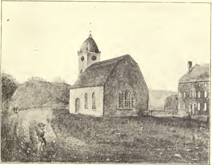
ST. PETER'S CHURCH, ERECTED IN 1714
