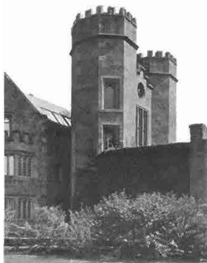
Looking from Weir Court to the northeast, Weir Hall on left, Weir Towers in middle – note, boarded-up windows. The secret courtyard wall goes from right to center
