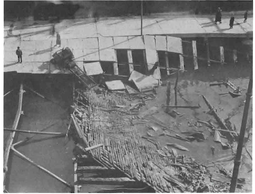
One of the docks that collapsed in Yokohama as a result of the earthquake. Photograph by Manly P. Hall.
