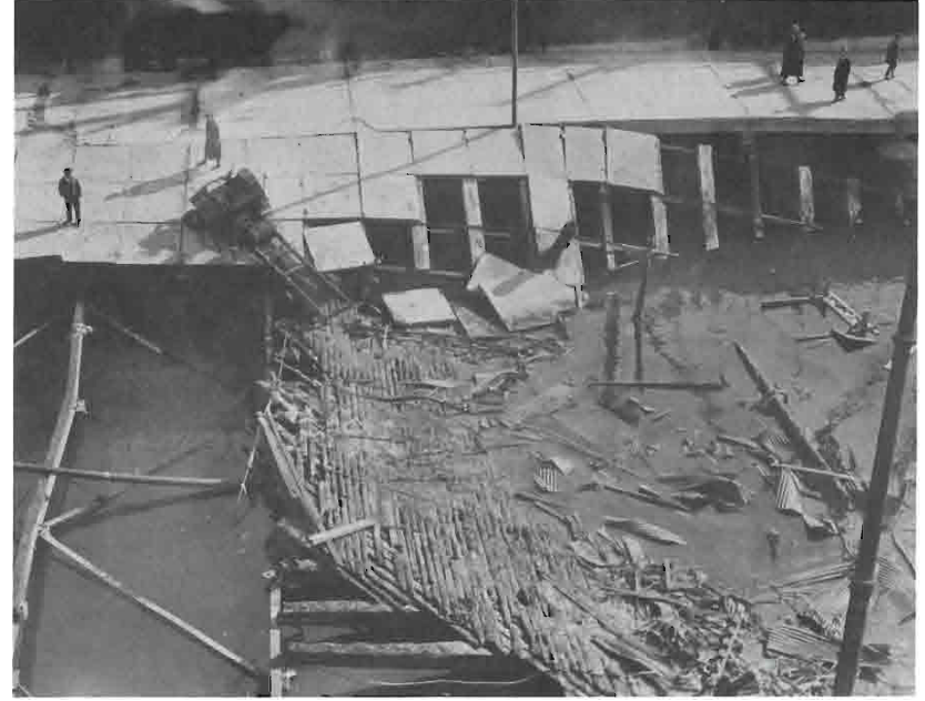
One of the docks that collapsed in Yokohama as a result of the earthquake. Photograph by Manly P. Hall.
