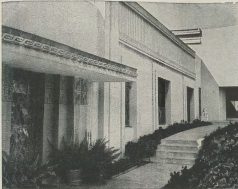
ENTRANCE TO THE BUILDING UNITS THAT NOW CONTAIN THE LIBRARY, THE BOOK BINDERY, STOCK ROOM, EDITORIAL ROOMS, PRINTING PLANT, AND THE GENERAL OFFICES
