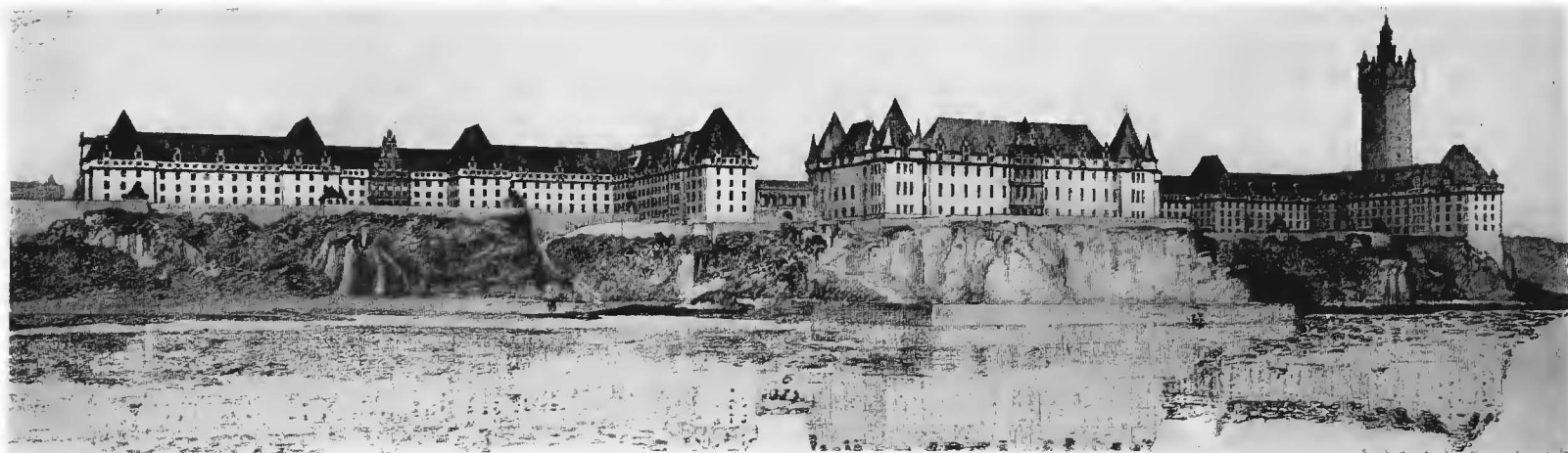
New Parliament and Departmental Buildings, Ottawa, Canada Dunn, Watson & W. Curtis Green, Architects
