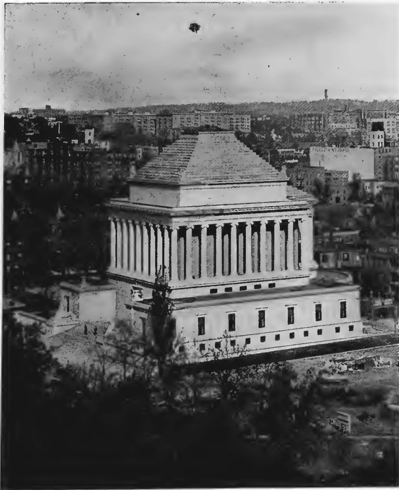
View of Building, Showing Solid Limestone Roof
