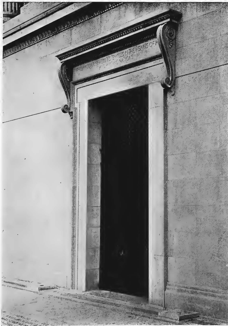
Detail View of Entrance Doorway
