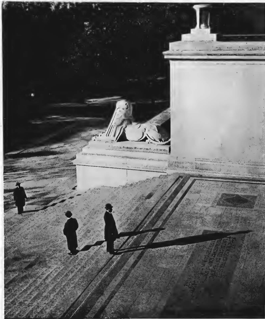
Forecourt, Taken from Top of the Side Pylon
