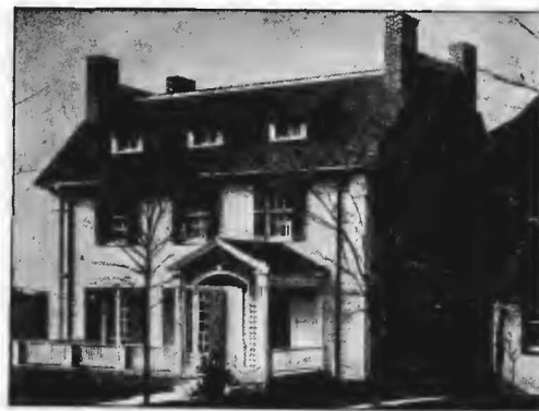
Walls finished with Cabot's Old Virginia White Roof finished with No. 346 Dark Gray Creosote Stain Walter Boschen, Architect, St. Joseph, Mo.
