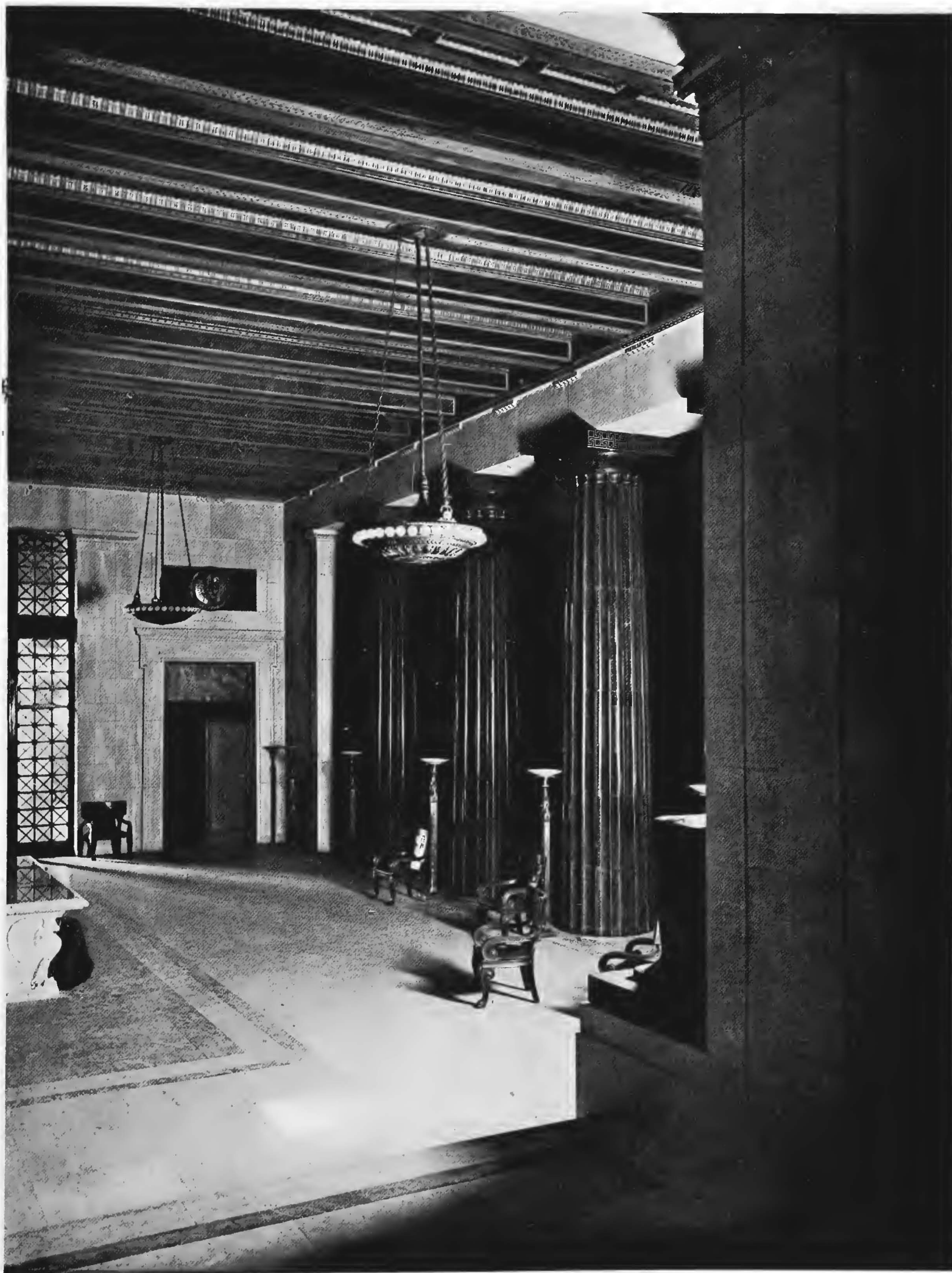
DETAIL VIEW OF ATRIUM TEMPLE OF THE SCOTTISH RITE, WASHINGTON, D. C. JOHN RUSSELL POPE, ARCHITECT
